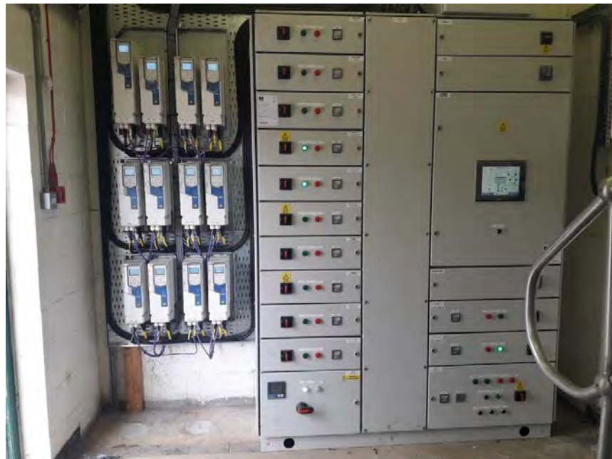
Upgrade works completed at Kentstown Wastewater Treatment Plant
