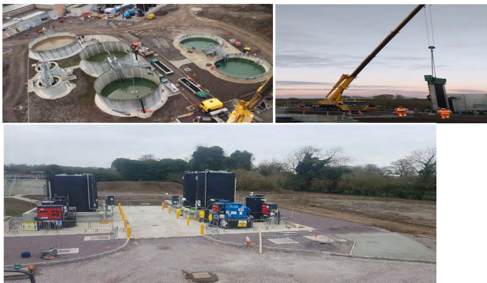
Upgrade works at Liscarton Water Treatment Plant , Navan.
