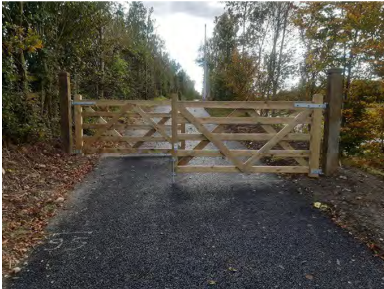
Kells By-Pass Footpath
