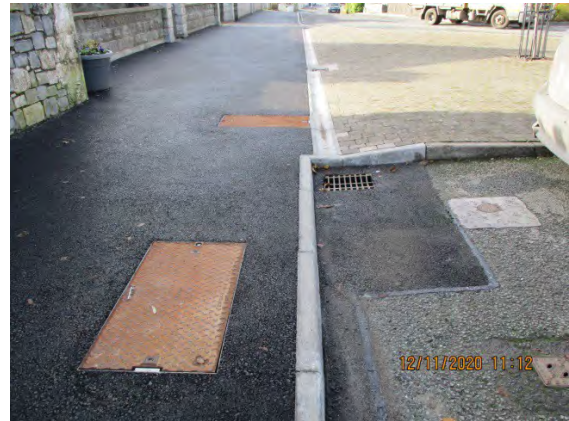
Longwood Footpath Works
