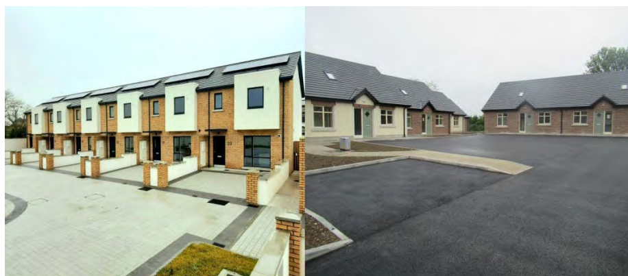
Direct Construction – Bettystown
