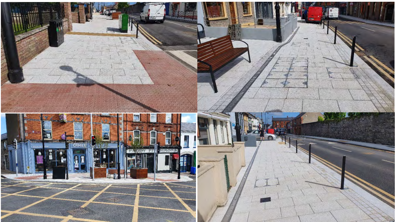
Works Completed on Railway Street
