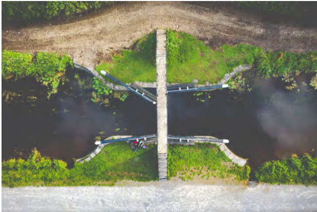
Royal Canal Greenway – Boyne Aqueduct
