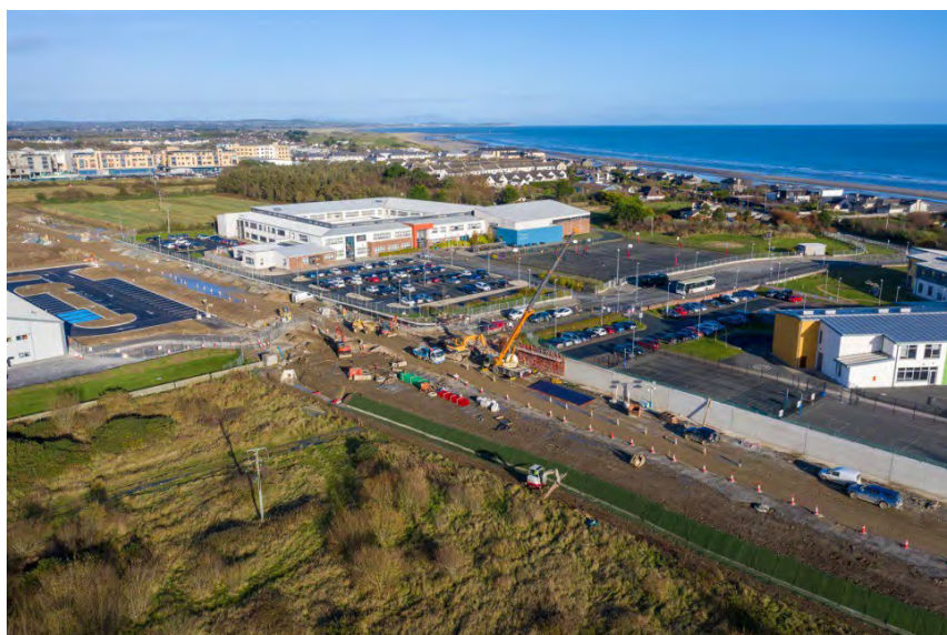
R150 Spine Road – Aerial Image of Construction
