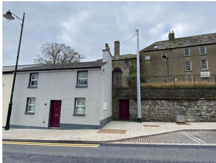
Works completed on Bridge Street
