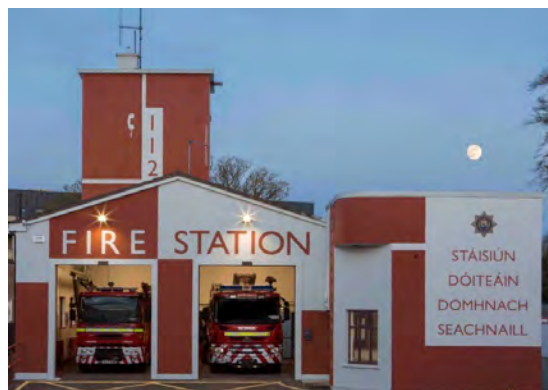
Dunshaughlin Fire Station following upgrade
