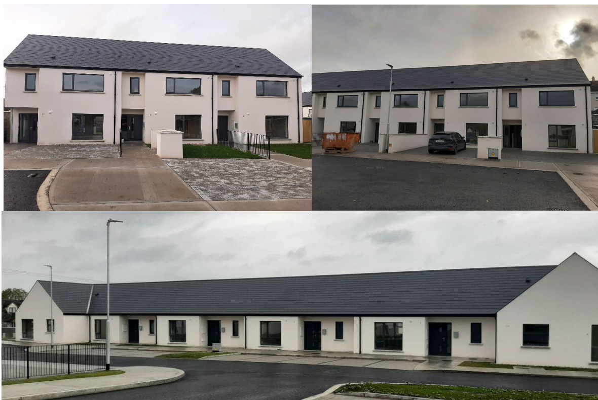
Meath County Council Site Direct construction – Staleen Park, Donore (€4m)
