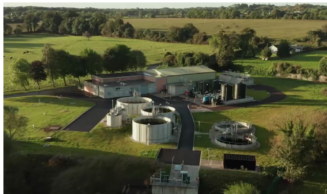
Liscarton Water Treatment Plant
