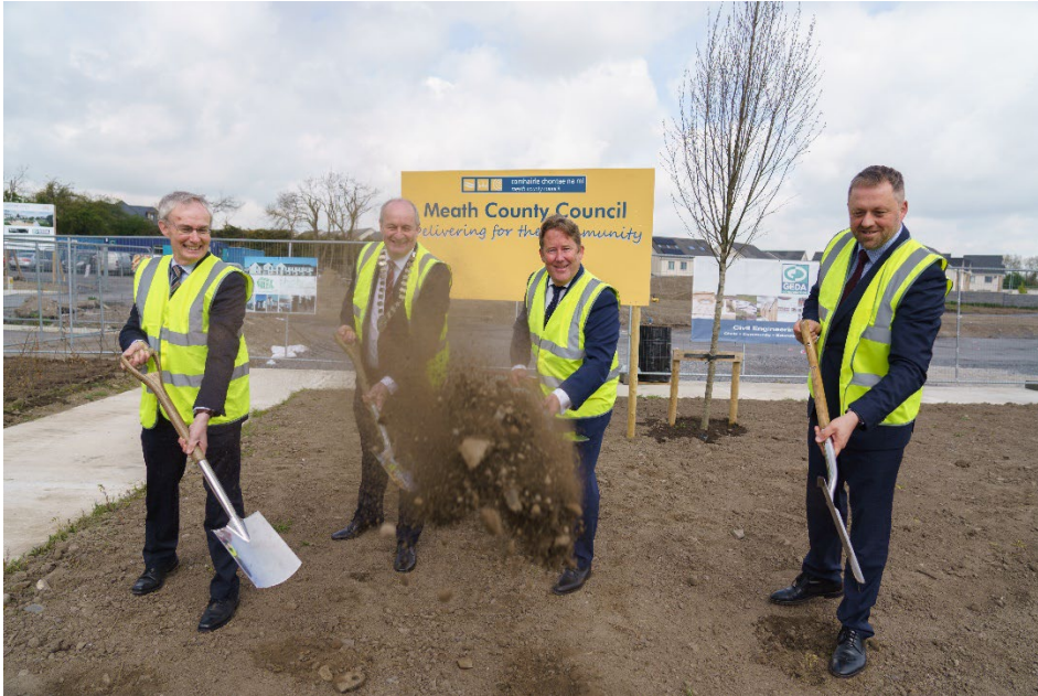
A sod turning ceremony led by the Minister for Housing, Local Government and Heritage, Darragh O'Brien, and supported by Cathaoirleach of Meath County Council, Councillor Sean Drew, Minister of State for European Affairs, Thomas Byrne TD and Deputy Chief Executive, Des Foley to mark the start of Phase 2 of works in Lagore Lawn, Dunshaughlin.
