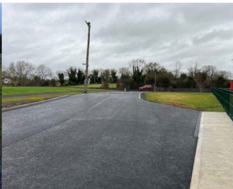
St. Brigids GFC – pictured after works
