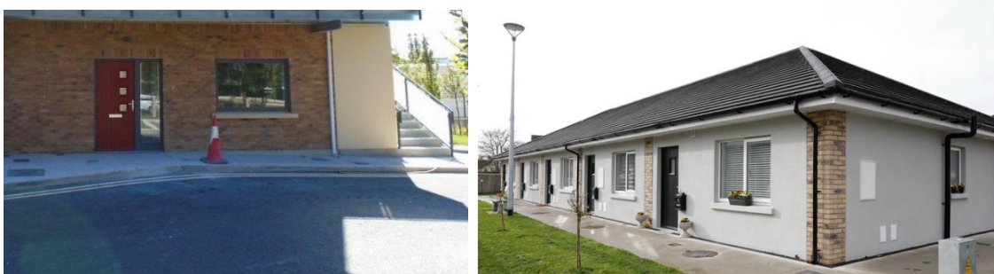
Level access units delivered through Part V and AHB Delivery (The Arches Dunshaughlin and Colliers Place, Duleek)
