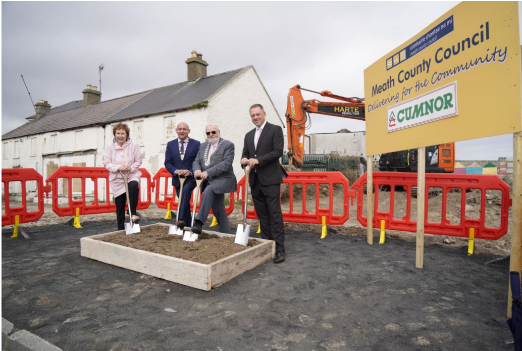
A sod turning ceremony to mark the start of the works on Bettystown Library took place led by Cathaoirleach of Meath County Council, Cllr. Nick Killian, Minister of State for European Affairs, Thomas Byrne T.D., Cathaoirleach of Laytown/Bettystown MD, Cllr. Wayne Harding and Chief Executive, Jackie Maguire.
