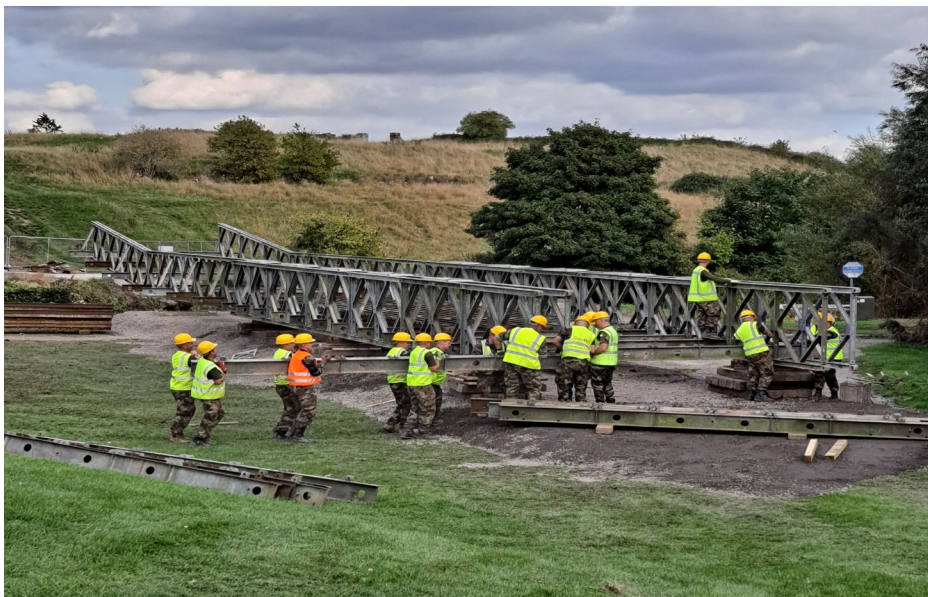
The temporary Bailey Bridge pictured being installed in Trim
