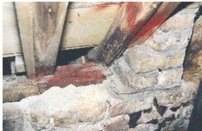
*Decayed wallplate and rafter showing timber to be cut back.*
