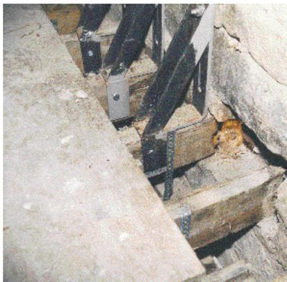
*Joist ends supported by steel brackets.*
