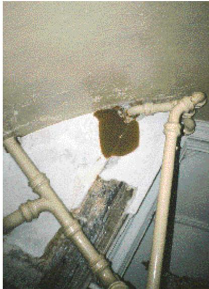
*Fruiting body on plaster caused by leaking pipe.*
