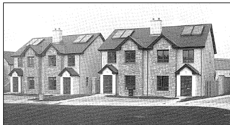
Timber frame, housing incorporating solar panels and heat pump system, Belmullet Co Mayo
