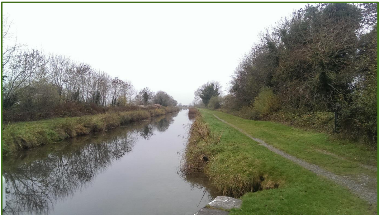
A section of the Royal Canal
