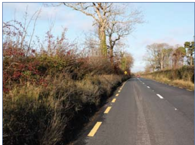
Figure 19 R157 Looking north towards CR571 Junction
