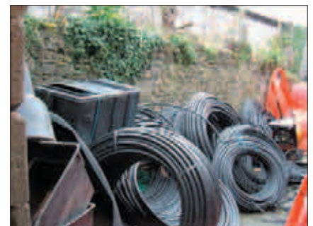
Materials piled against walls
