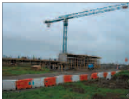
Construction site to west of town wall
