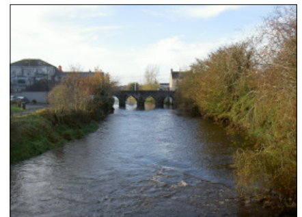
View north-west from footbridge towards Trim bridge
