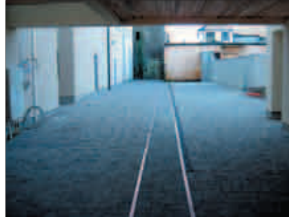
Line of wall delineated in paving at commercial development
