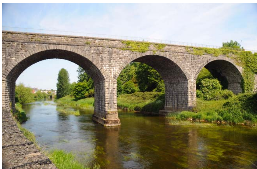
Protected view of the Railway Viaduct
