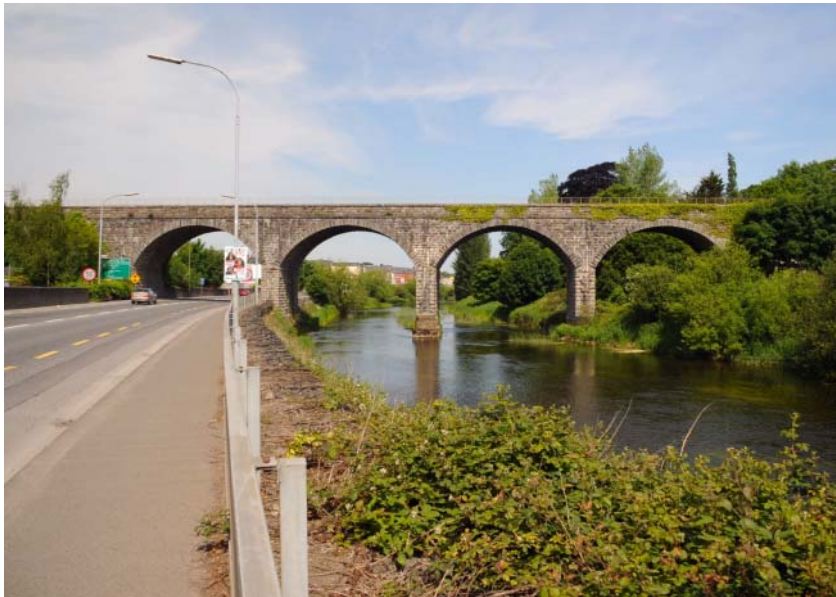
Navan Railway Viaduct (1850)
