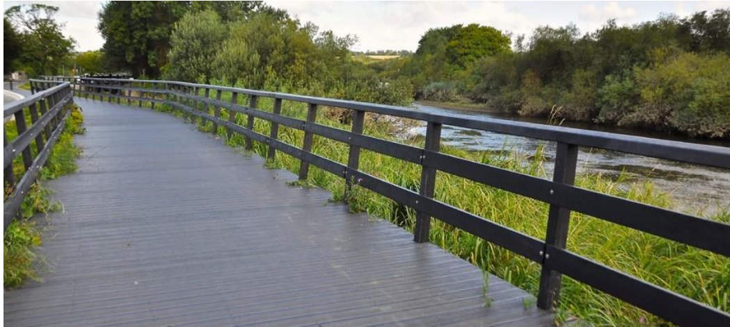
Figure 1.4 Boyne Greenway Upstream Recycle Plastic Elements Construction
