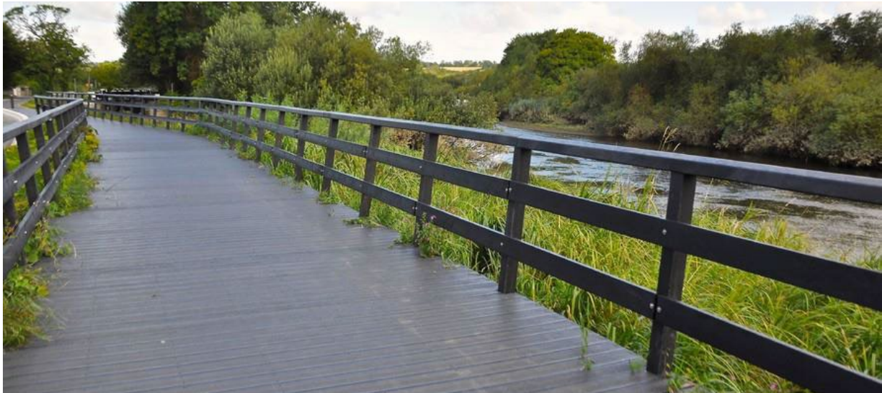
Figure 1.3: Boyne Greenway Upstream Recycle Plastic Elements Construction.
