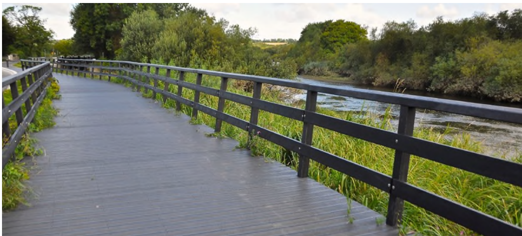
Figure 3 Boyne Greenway Upstream: Recycled Plastic Elements Construction
