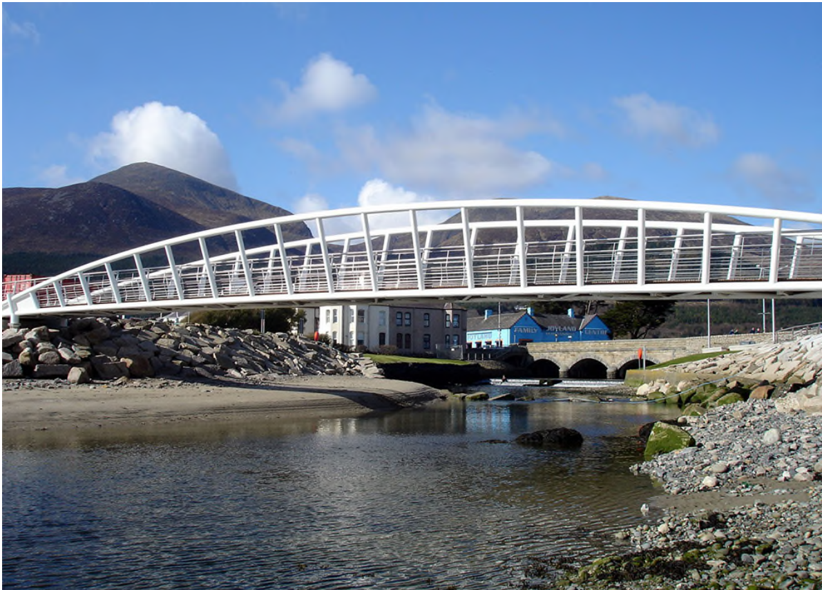
Figure 4 Typical Prefabricated Steel Arch Bridges
