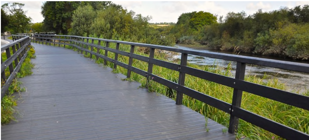
Figure 3 Boyne Greenway Upstream Recycle Plastic Elements Construction
