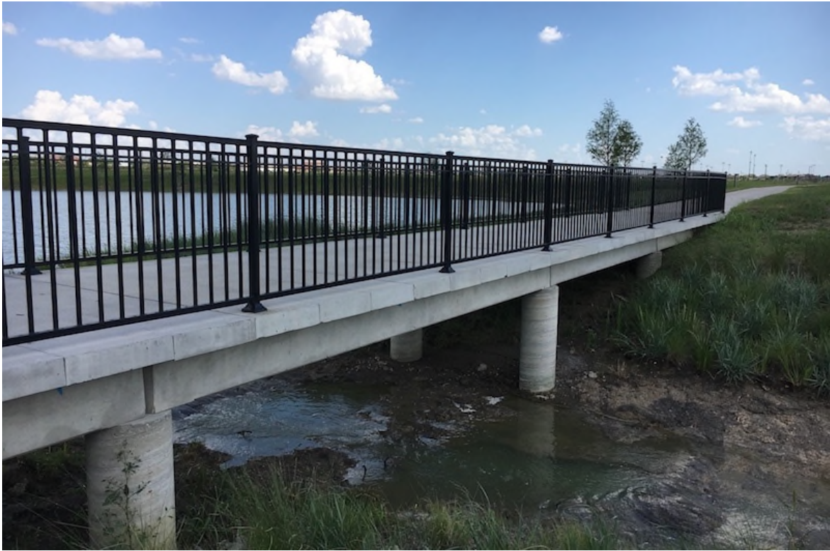
Figure 5 Typical Precast Concrete Bridges
