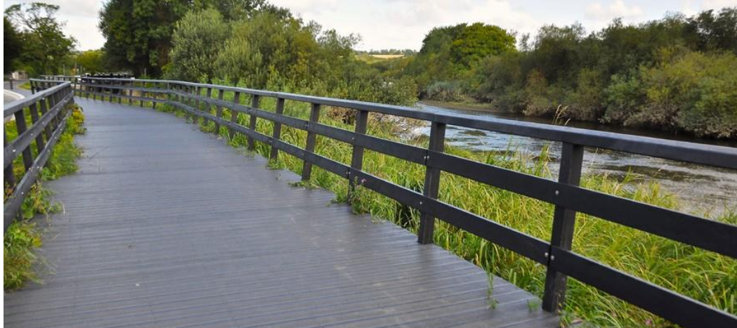
Figure 1.4 Boyne Greenway Upstream Recycle Plastic Elements Construction
