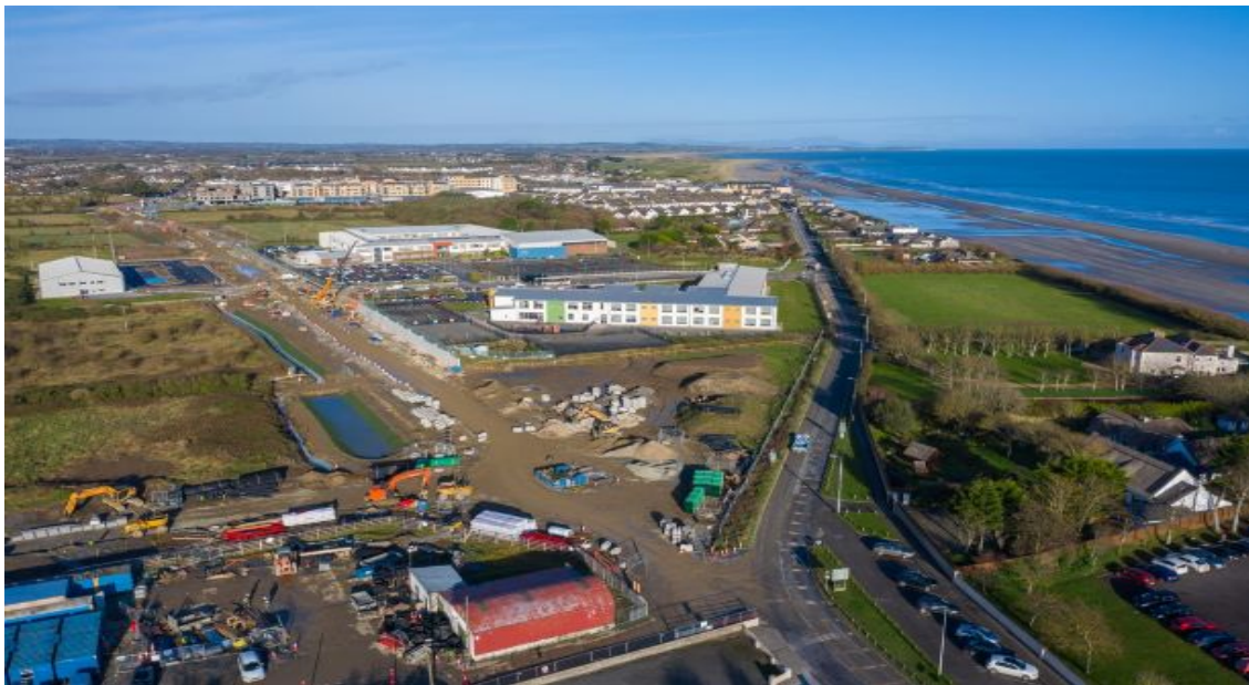
Work progressing on the R150 Laytown to Bettystown Spine Road
