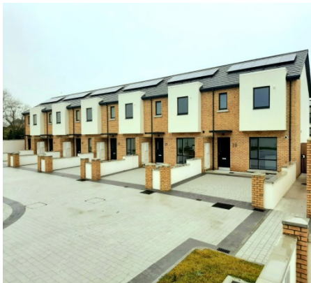
Direct Construction – Bettystown
