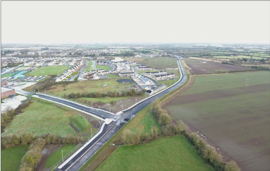
RORR School Road Junction looking north to R125
