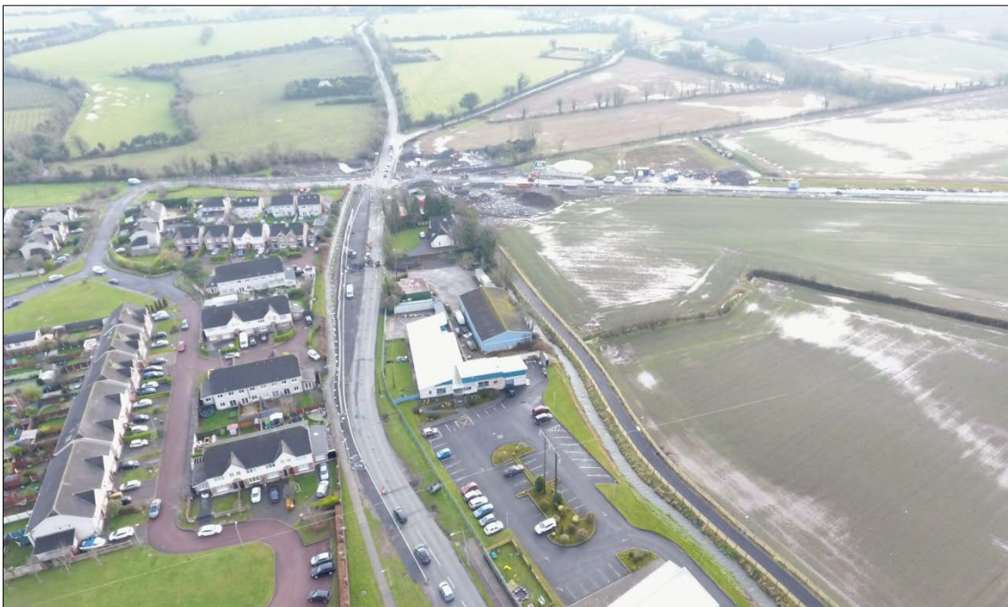
R125 looking east (Moulden Bridge estate on the Left, RORR on the right)
