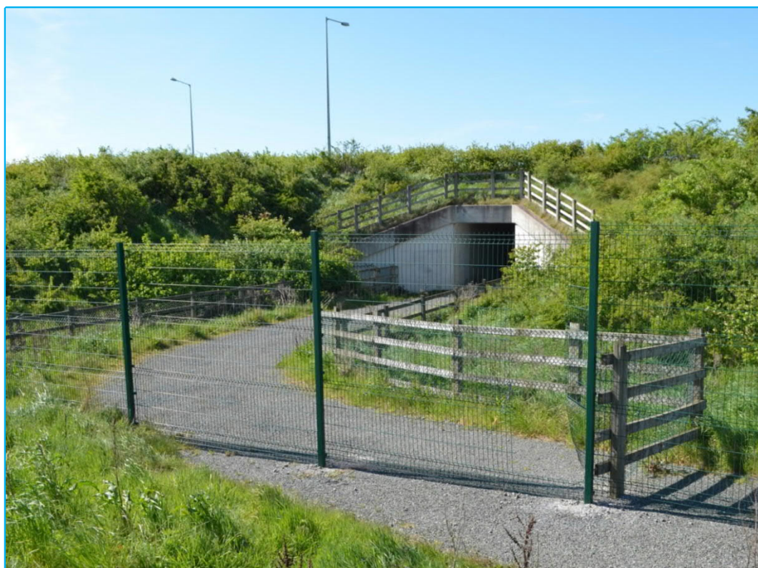
Figure 4.6. Blocked Access to Pedestrian/Cyclist tunnel under R157
