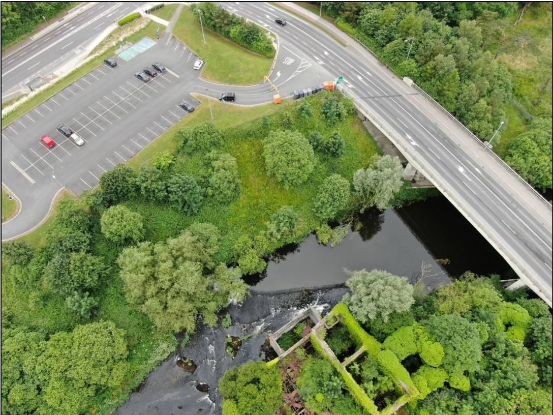
Figure 15: Bridge over the Blackwater and Carpark
