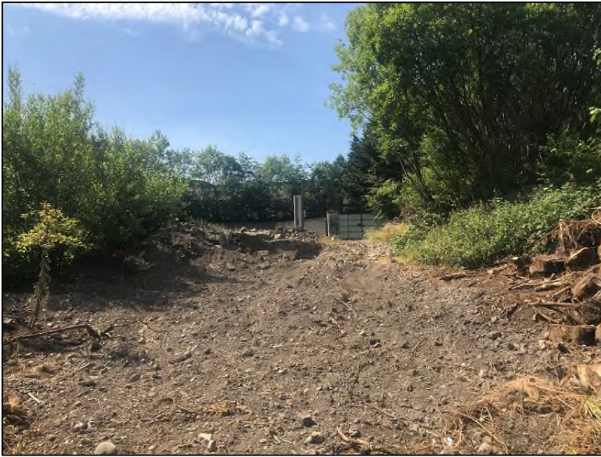
Figure 7: Recently disturbed habitat at compound
