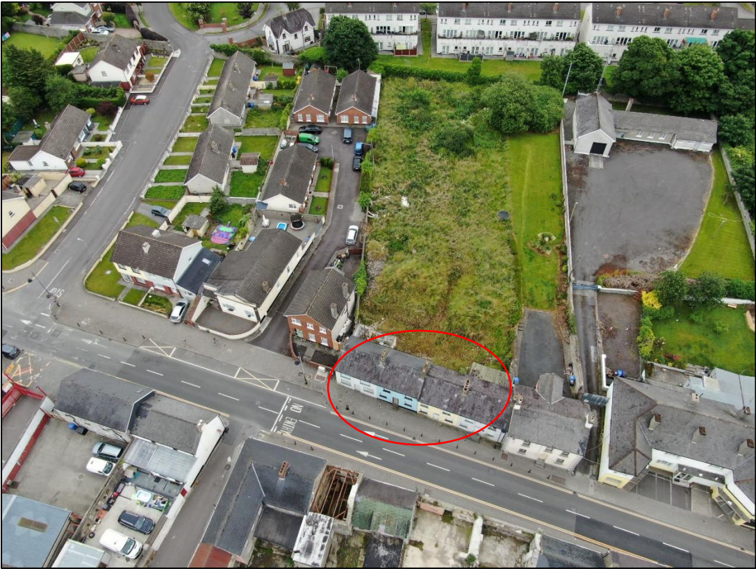
Figure 21: Example of derelict buildings on Flowerhill
