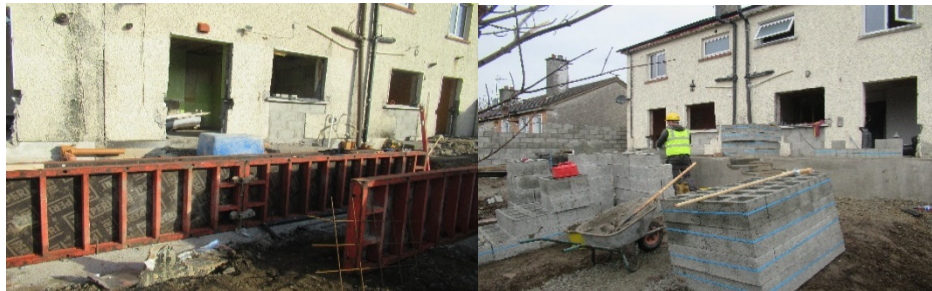
Refurbishment works commence in Alverno Court, Laytown
