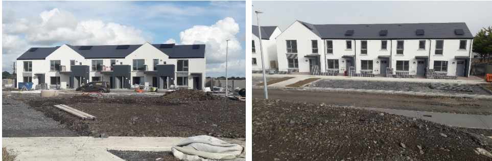
Meath County Council Site under construction – Lagore Road, Dunshaughlin (€5.8m)
