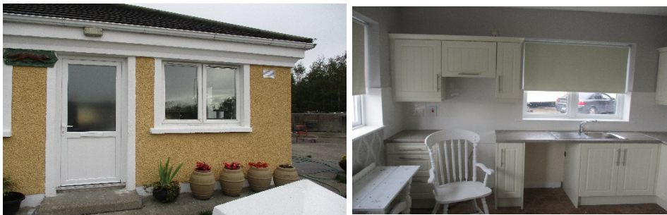
Upgrade Works St Patrick's Park Halting Site, Navan
