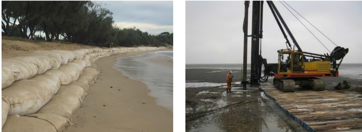
Figure 4-3 Typical Geotextile Filled Bags and Timber Piling Mat (Temporary)
