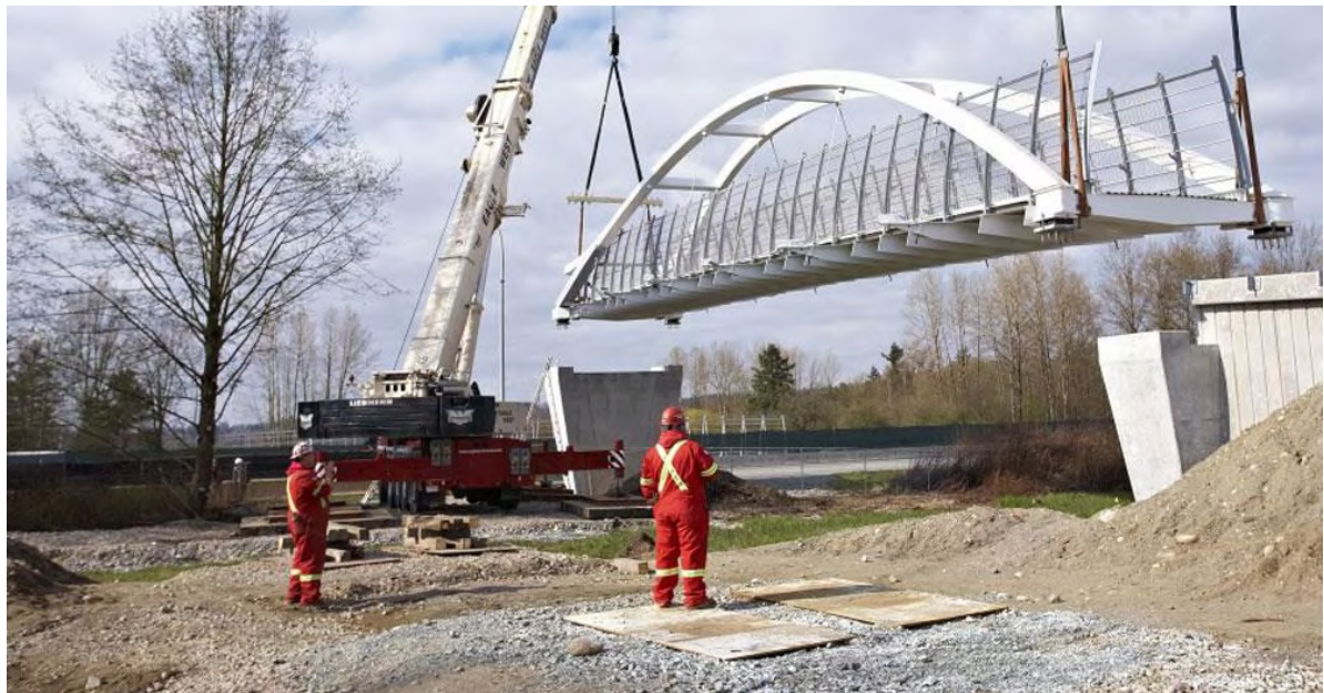
Figure 4-5 Typical Bridge Lifting Operations (One Lift)
