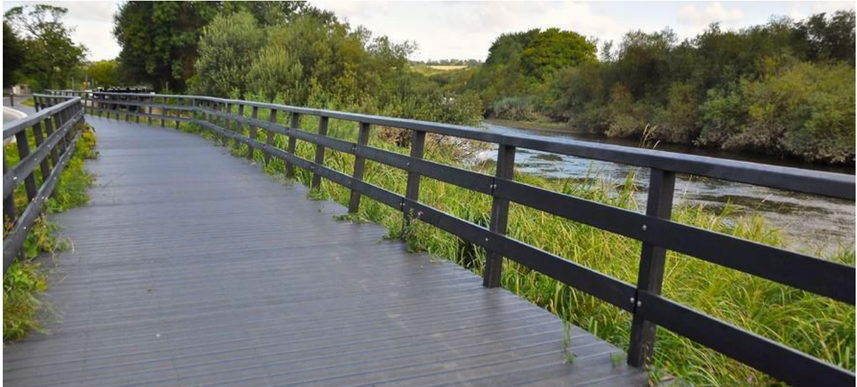
Figure 1.3: Boyne Greenway upstream recycle plastic elements construction.
