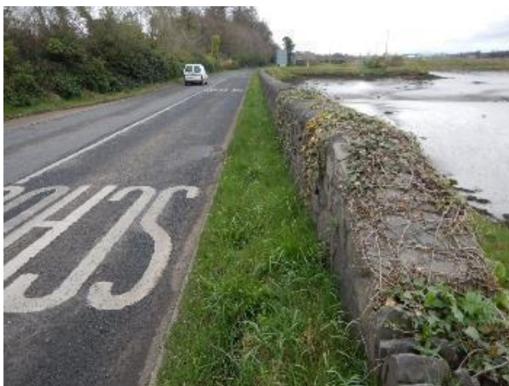
Figure 4.1: Regional road R150 with grass verge and wall in the foreground and mud flats in the background.
