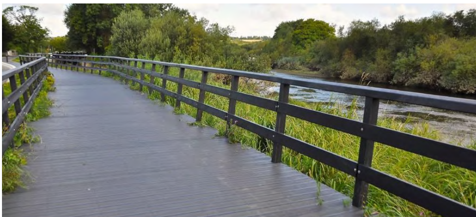
Figure 3 Boyne Greenway Upstream Recycle Plastic Elements Construction
