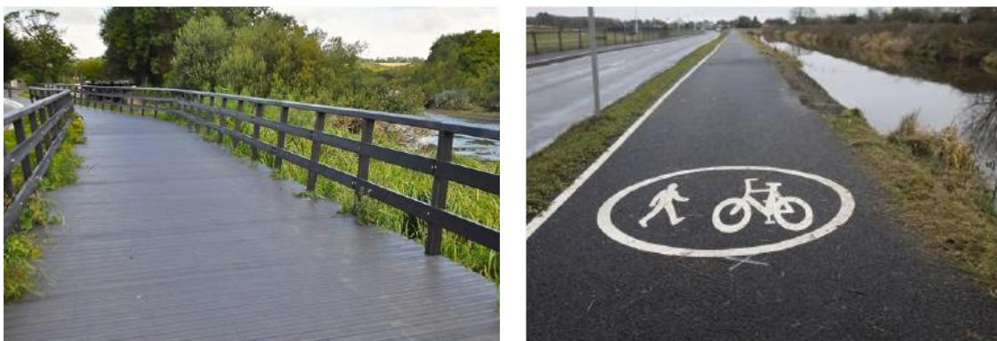
*Figure 1-2 Typical Greenway on Boardwalk and as a Bituminous Surface*
