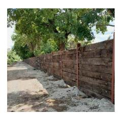
As part of the construction of the Navan to Kingscourt Greenway, rather than dispose of old rail sleepers the Council has utilised them to provide screen fencing to adjacent properties.
