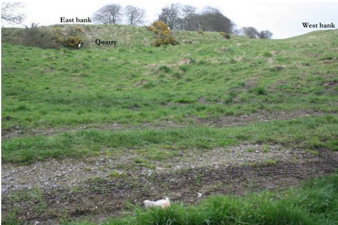
Fig. 53 Surface erosion, tyre tracks and discarded dog litter bag at the northern end of Tech Midchúarta (April 2018).
