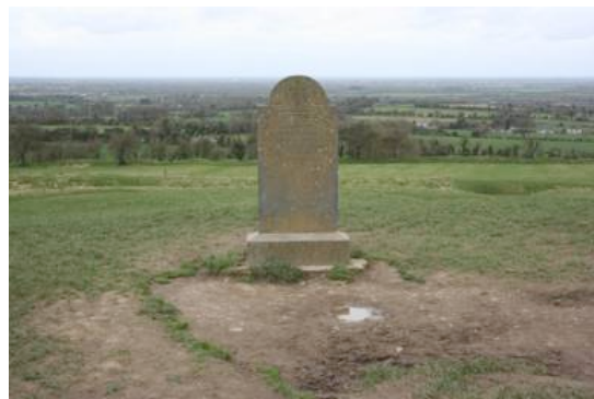
Fig. 24 Erosion and surface water around the 1798 memorial on the summit of the Forrad (April 2018).
