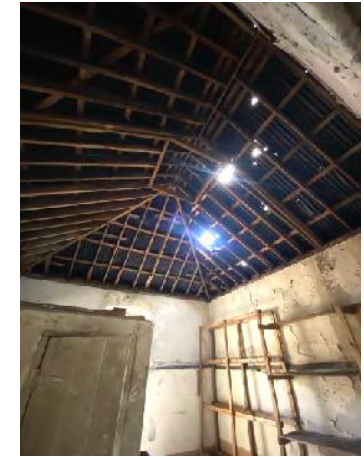
05: Timber roof structure of extension to East.
