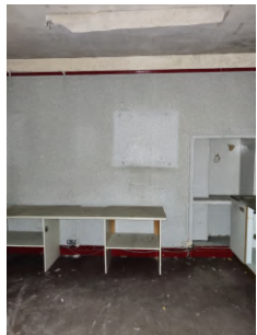
10: South-East room on GF looking North. R.0.B2
