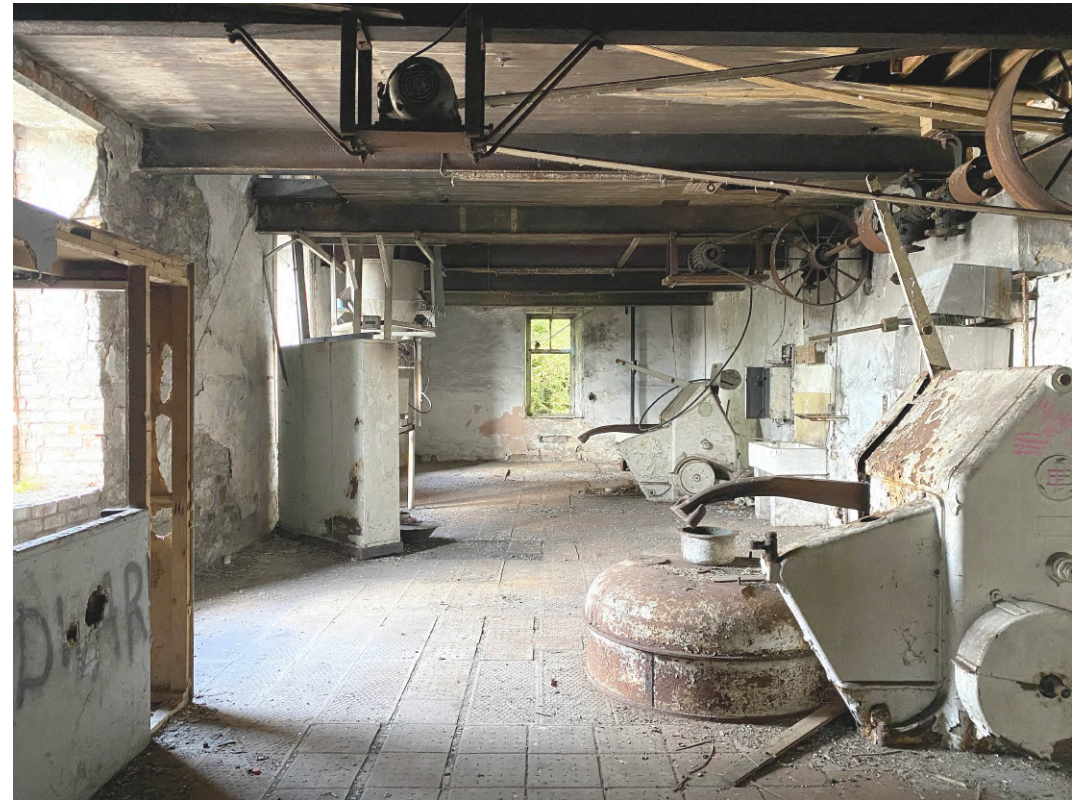
Photograph: Current condition of Spicer's Bakery on first floor looking north
