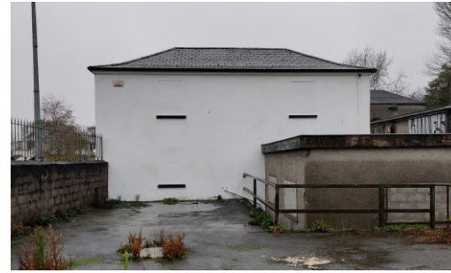
04: West Elevation with existing windows blocked and adjoining single storey extension.
