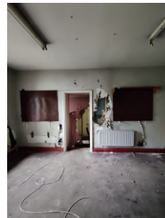
13: North Room leading to rear extension. R.0.B3
