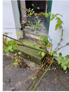
03: Side door entrance to East Elevation.
