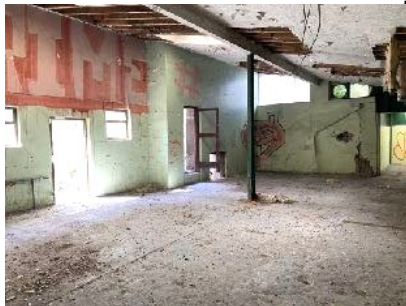
07: Recent extension building
