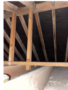
16: Existing roof space condition.
