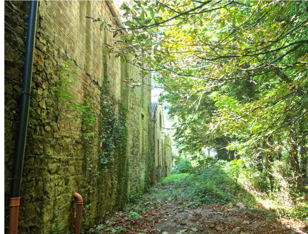
Site Photo of Rear Boundary (2022) Architect's Own
