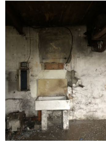
04: Eastern Wall with infilled openings from original 4 storey mill building.
