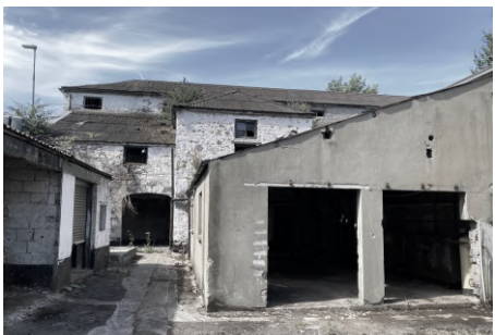
06: Courtyard Context looking towards Mill building.
