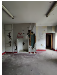
12: North Room looking towards front elevation. R.0.B3
