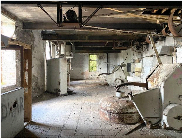
01: Original Mill/Bakery work space looking North, showing 3 storey conversion for bakery use: Bakery machinery remains in-situ.
