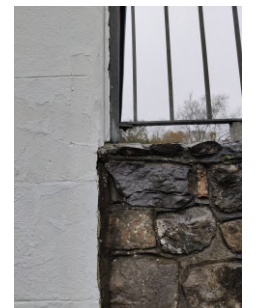
10: Connection to stone site wall to East of existing office building.
