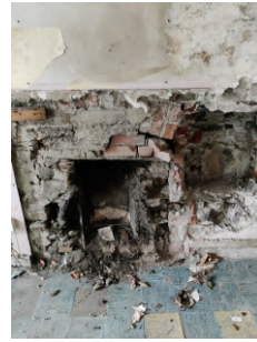
05: Fireplace to north wall in living area. R.0.B1
