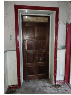
06: Internal view of front door.
