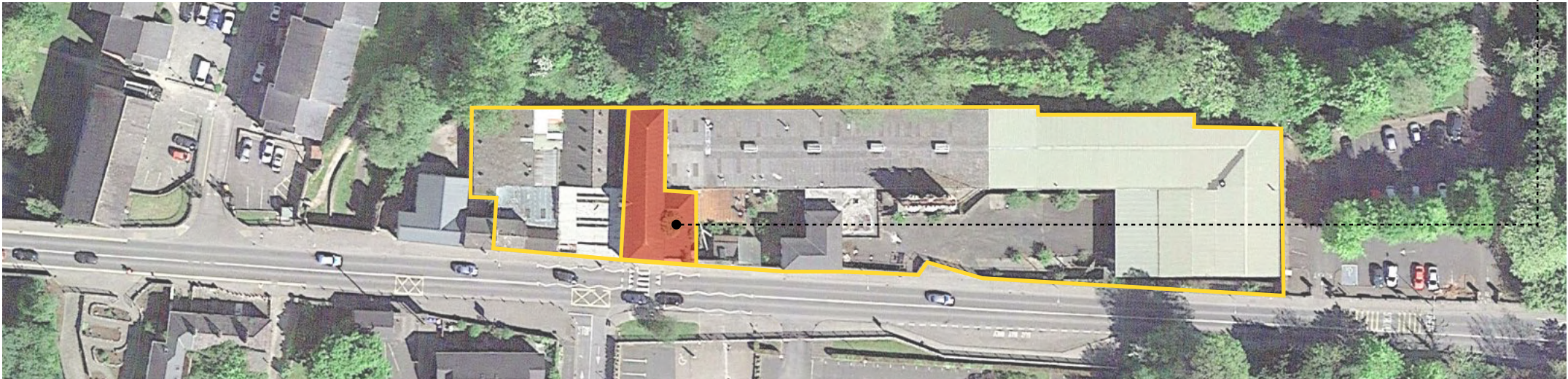
Aerial view of existing structures
