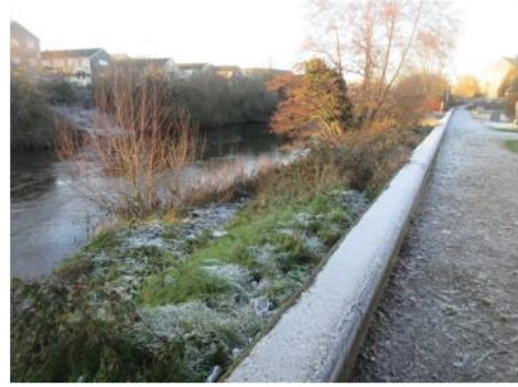
Area of infilled Dry Dock [48] facing S
