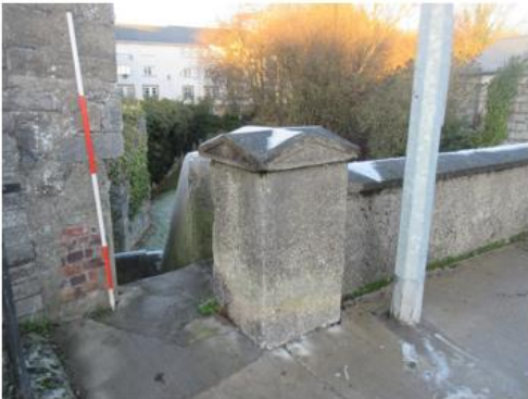
Somerville Bridge [23] and Step Access [24]
