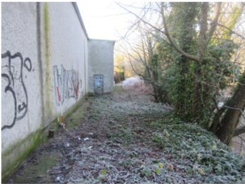
Northern wall of Buildings [54]
