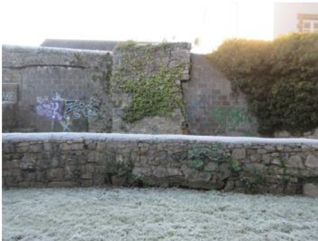
Blocked gate [25], Building wall [26] and modern wall
