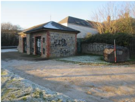
Water Pump House [50]
