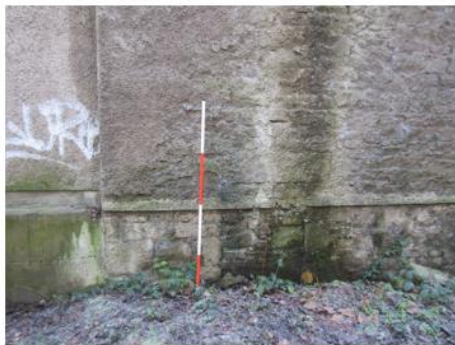
Blocked Door [18] in Wall [13]
