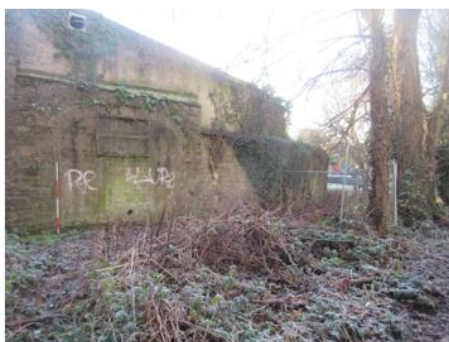
Wall [1], Gate Arch [3] with Extension [2]
