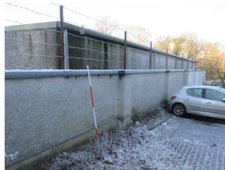
Buildings [54] from carpark [57]
