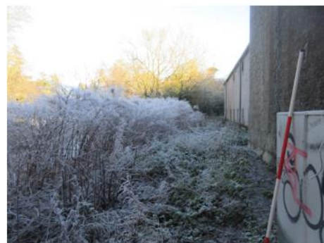
N wall [19] from Buildings [54]
