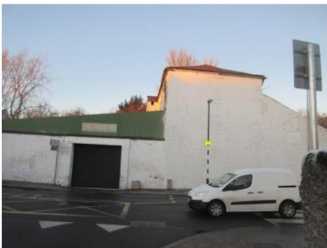
Infilled windows to Building [11]
