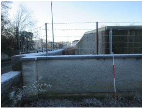
Buildings [54] from carpark [57]
