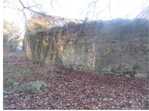
Curving boundary Wall [1]
