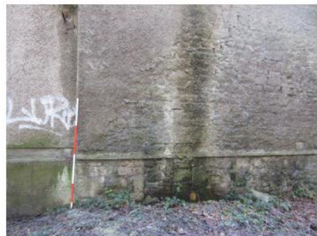
E end of Wall [13] with blocked door [18]
