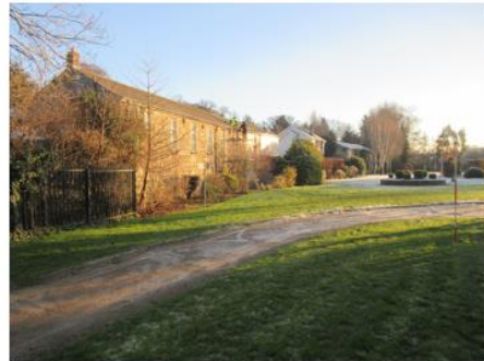
Building [41] with infilled Navigation [40]
