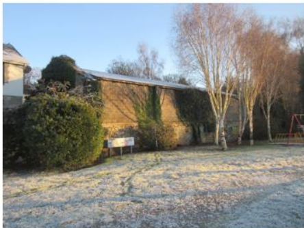
Wall [45] and infilled canal channel
