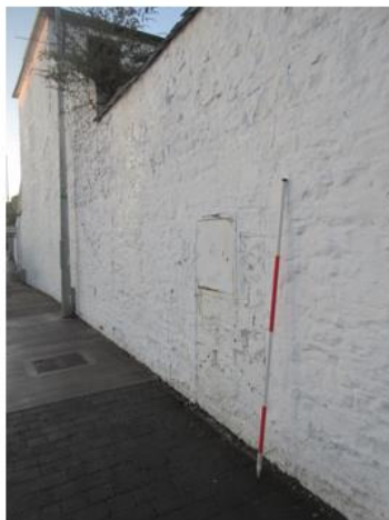
Boundary wall to building [35]
