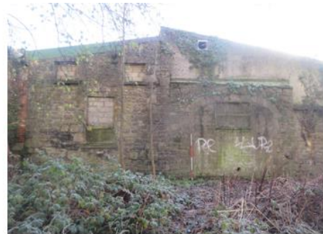
Gate Arch [3] and Building [4] with Extension [2]
