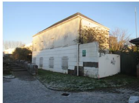
Extension building [51] to Buildings [53]
