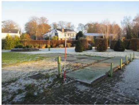
Water pumping station [50]
