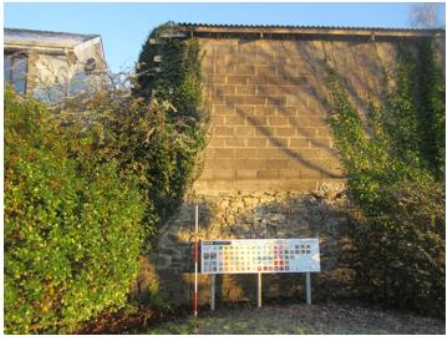
Building ruin [44] and Wall [45]
