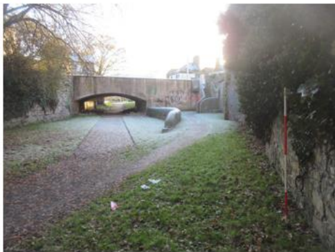
Infilled Canal [32] facing Somerville Bridge
