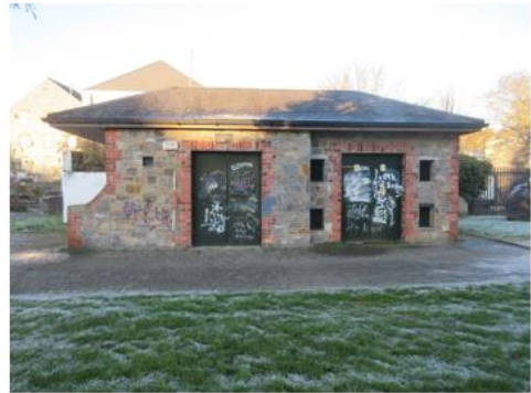
Water Pump House [50]
