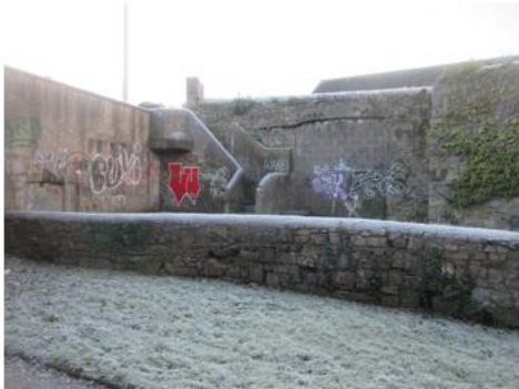
Somerville Bridge [23] and step access [24]
