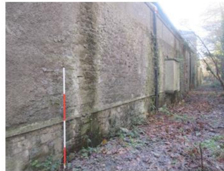
Blocked Door [18] in Wall [13]
