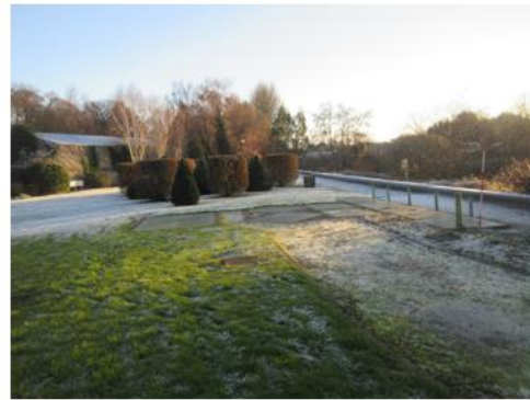
Water pumping station [50]
