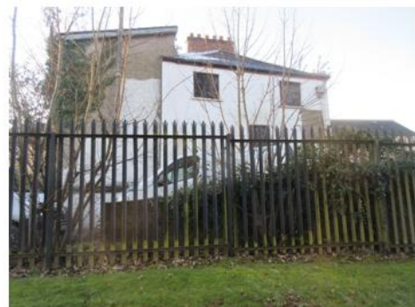
Buildings [53] with extension
