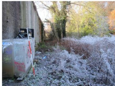
N wall [19] from Buildings [54]
