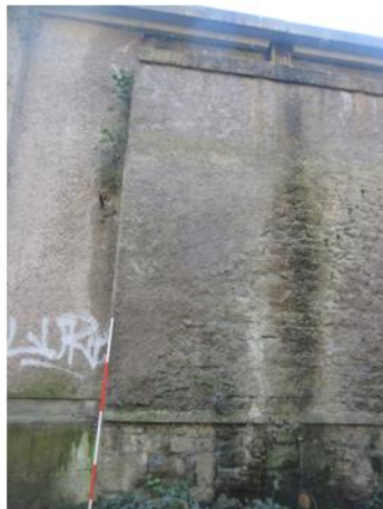
E end of Wall [13] with blocked door [18]
