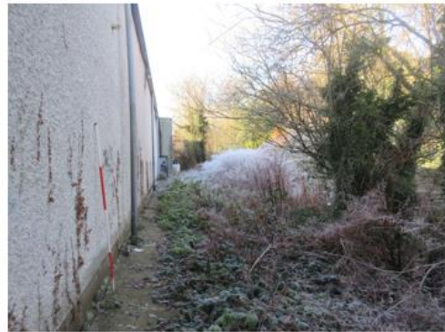
N wall [19] from Buildings [54]
