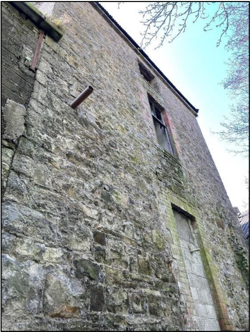
Figure 26: Derelict stone building at Spicer's Mill site (BL1)
