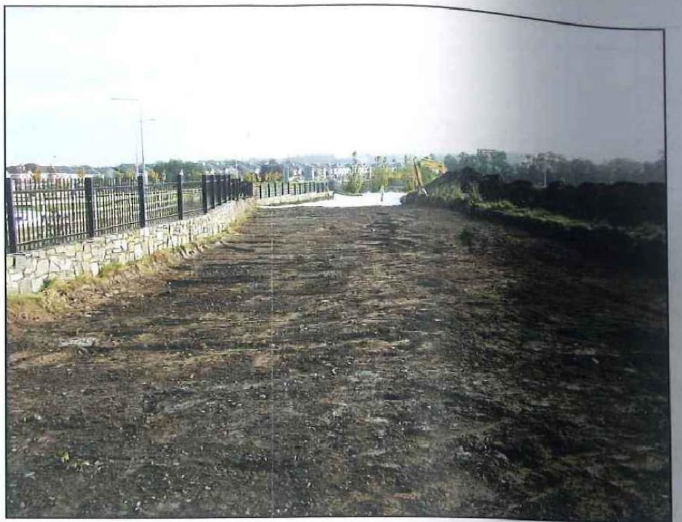
Plate 2 Placing of terram over stripped area prior to importation of stone
