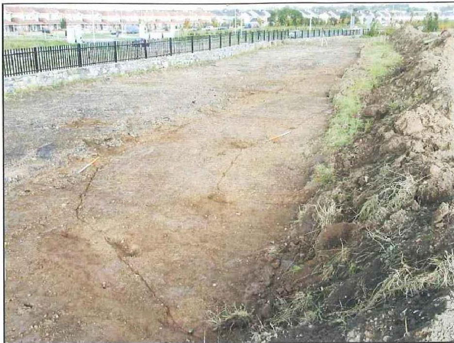
Plate 1 Topsoil removal along Area A. Ditch C295. Looking northeast Topsoil stripping in advance of the haul road along the northern side of the site
