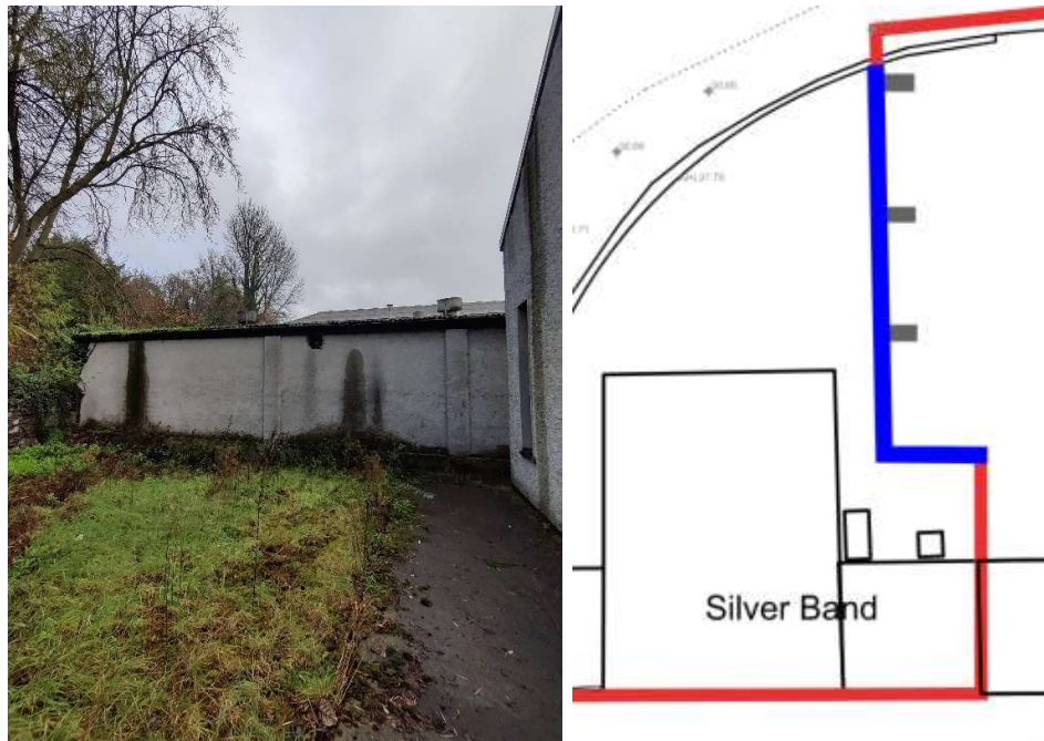
Figure 4.3-Existing Boundary Wall and Possible Buttressing Arrangement
