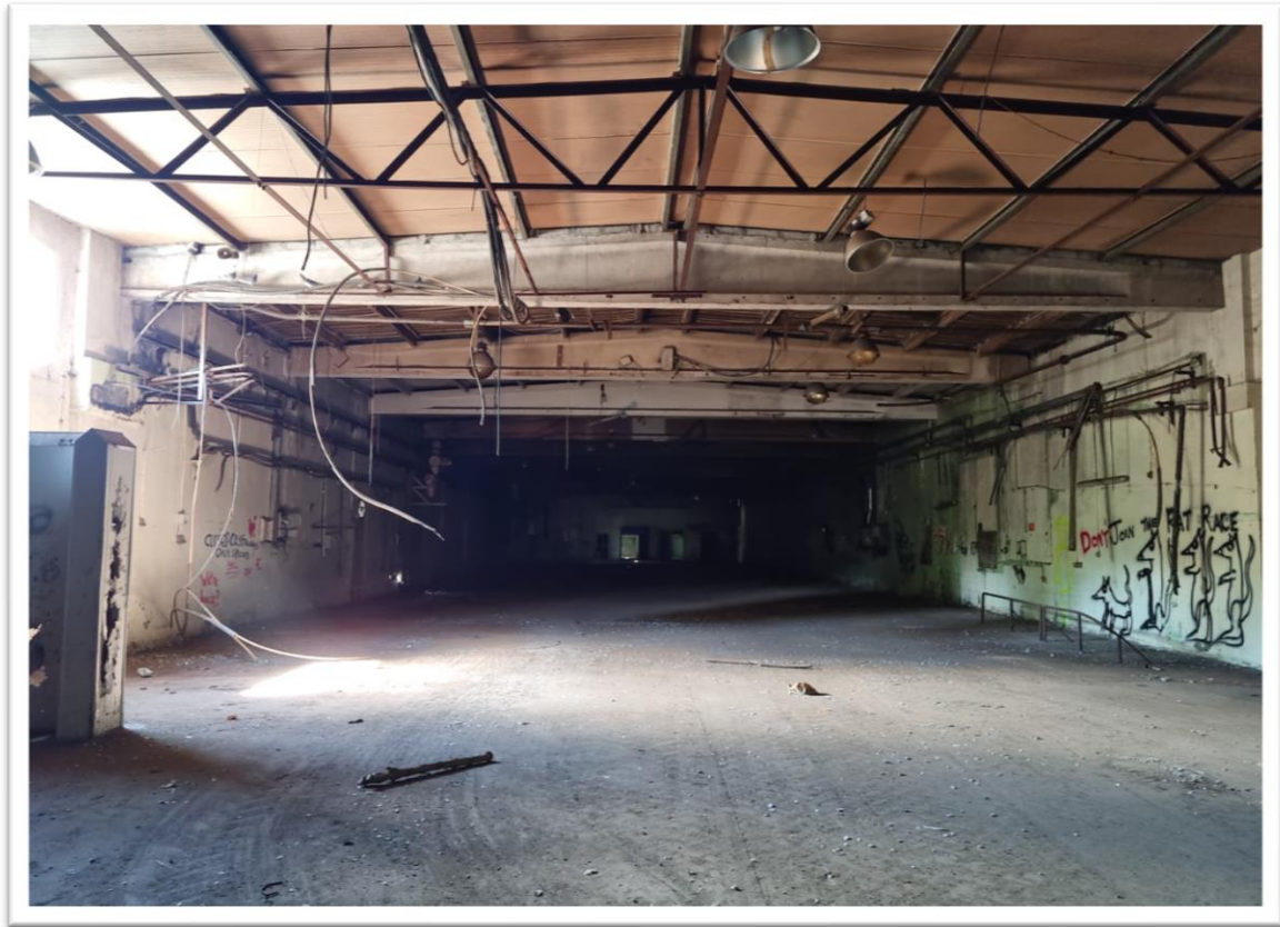
Interior of warehouse
