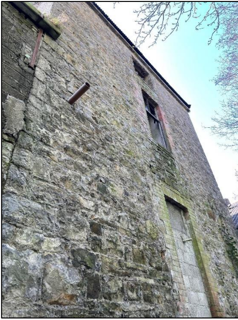
Figure 18: Derelict stone building at Spicer's Mill site (BL1)
