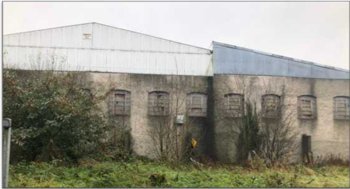
Figure 10 Vacant Structure formerly used for NCT Testing
