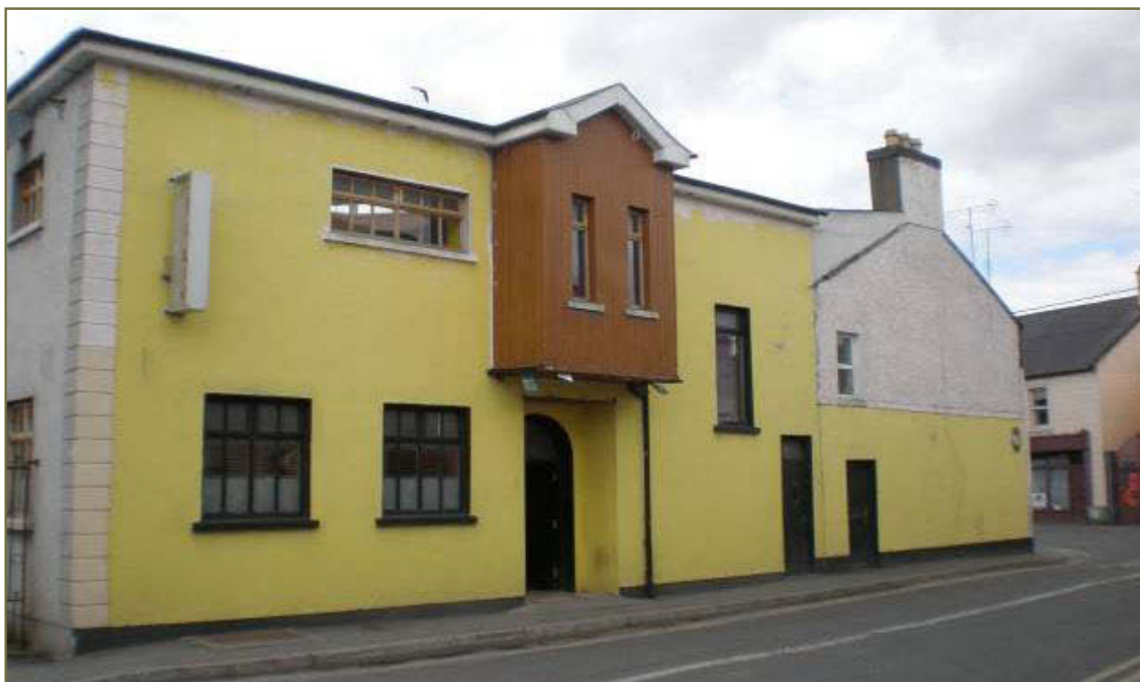
Fig.12: Modern developments at the junction of Connaught Street & Main Street.
