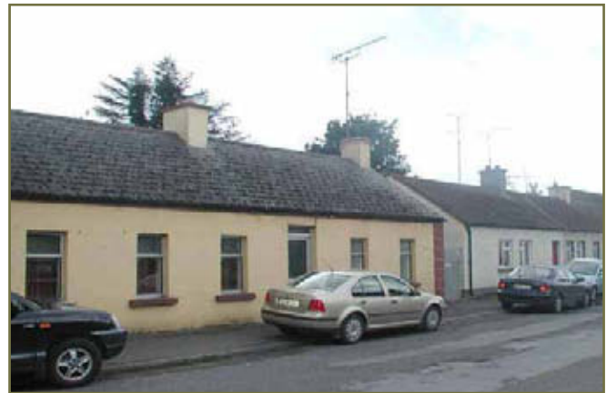
Fig.11: Modest vernacular houses on Connaught Street with their windows, doors and roofs replaced with modern materials.
