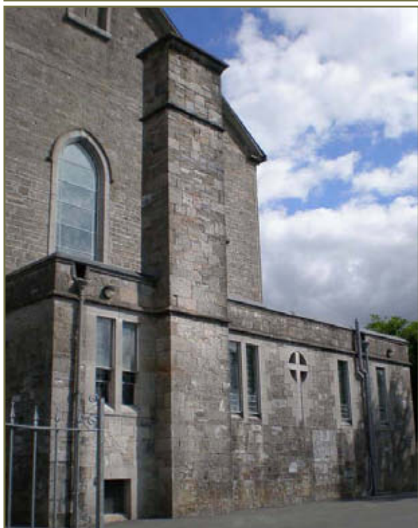
Fig.2: Cast-iron water-pump on Connaught Street & the sacristy to the rear of St James's Catholic Church, two protected structures outside the current ACA boundary for Athboy.
