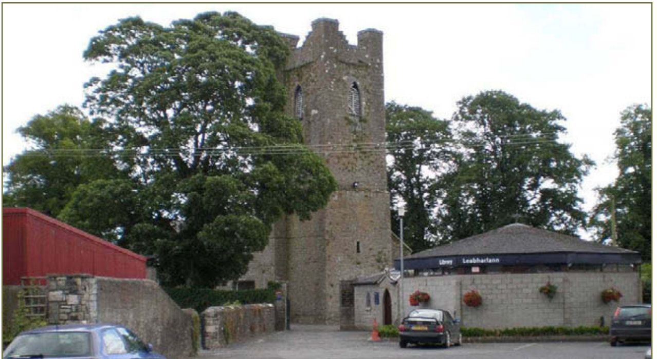
Fig.20: Norman tower of St James's Church of Ireland and the former sexton's house with library extension at the entrance to the church grounds.
