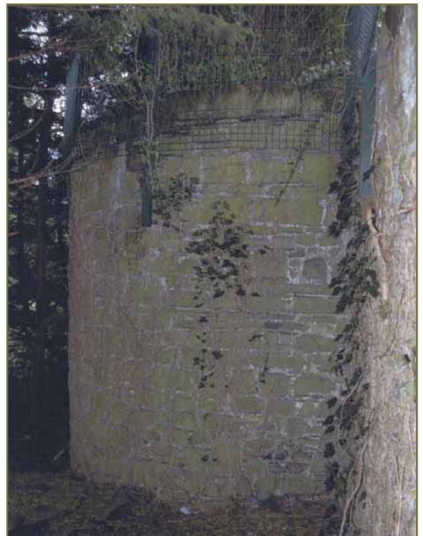
Fig.3: Semi-circular cut-stone bastion to the south of the town, part of the remains of the extant walls of Athboy.
