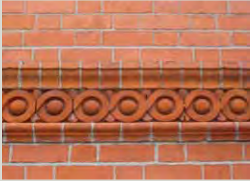
A example of the decorative use of moulded brickwork and terracotta in a stringcourse
