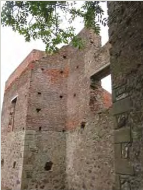
Mountjoy Fort, Co. Tyrone, built c. 1603, is the earliest known surviving Irish building where brick was used as the substantive building material for walls
