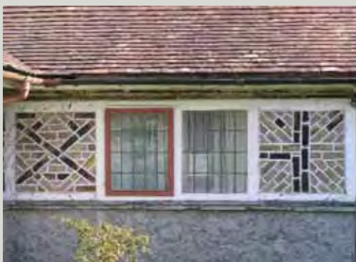
The Arts and Crafts Movement in the late nineteenth century promoted the use of handcrafted building materials, including handmade bricks, as in this example of a house at Talbot's Inch village, Co. Kilkenny designed by the architect William A. Scott and built 1896-1904
