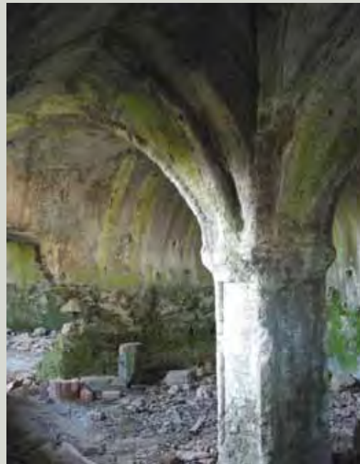
The brick-vaulted undercroft of Jigginstown House, Co. Kildare
