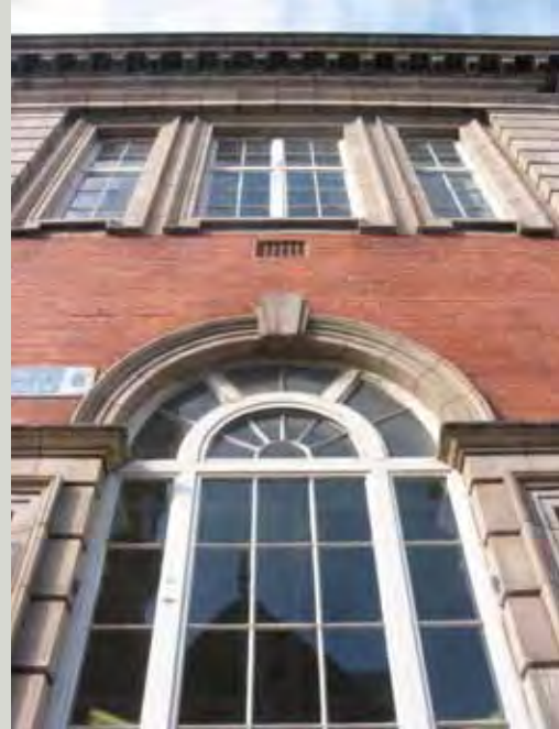
Rathmines Library, Dublin, opened 1913, constructed of Arklow brick and terracotta designed to resemble stonework
