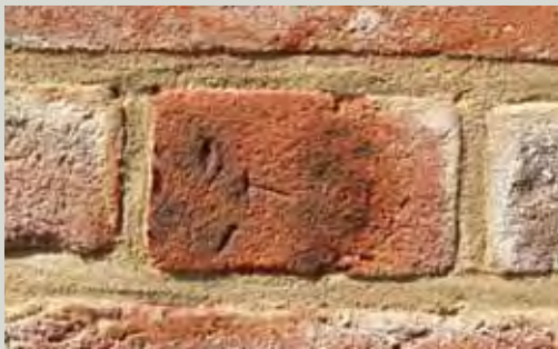
Remedial work in the form of a quality pigmented mortar repair. It shows that, when necessary, and executed with great skill, a mortar repair can provide a temporary repair that achieves the desired effect
