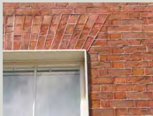
A typical Irish eighteenth-century flat arch window head. It differs from similar English flat arches of the period in that the arch does not splay widely at either end
