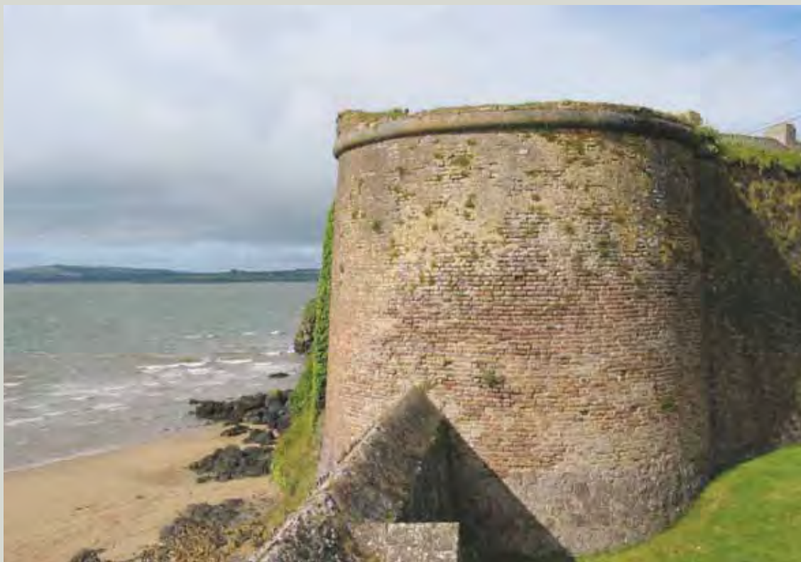
Duncannon Fort, Co. Wexford was partly repaired and rebuilt in Flemish bond brickwork during the eighteenth century
