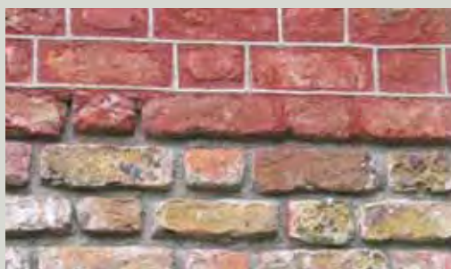
Tuck pointing in practice
