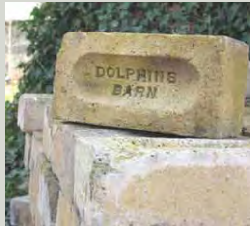
Machine-made brick from the Dolphin's Barn Factory in Crumlin dating from the early twentieth century is recognisable from its distinctive yellow colouring and the manufacturer's name impressed into the 'frog' or indentation in the bed face of the brick
