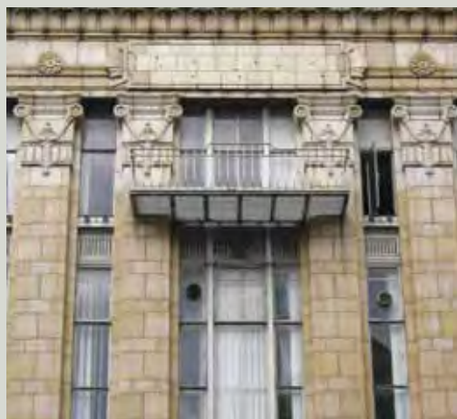
Burton's, Dame St, Dublin, designed in 1929 by Harry Wilson, is an example of high quality faïence cladding used to form a giant classical order to the façade
