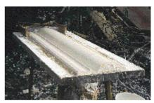
Reverse mould showing template and horse in position.
