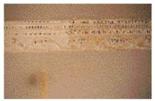
Cleaned cornice on left contrasting with portion on right, which is obscured by layers of paint.
