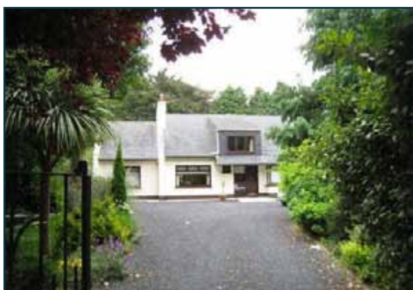
Fig. 25: Private house to the east of the Catholic church
