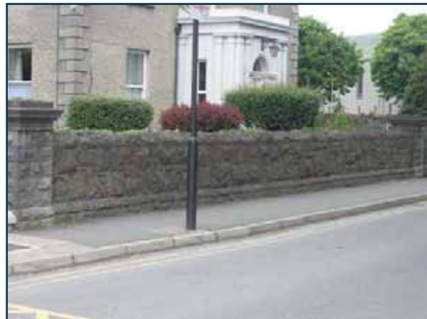
Fig.9: Rock-cut limestone wall
