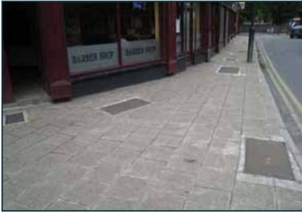
Fig.41: Profusion of service access in paving
