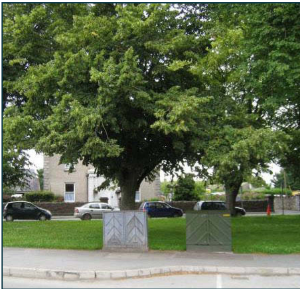
Fig.42: Service boxes in important views
