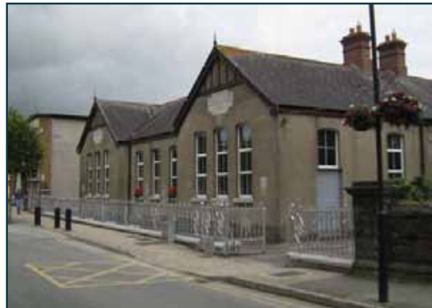
Fig.10: Metal railings to National School
