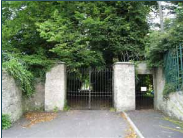
Fig.15: Entrance gates to St.Peter's church grounds
