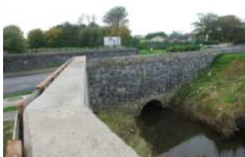
Flood defence wall and culvert parapet in Mornington East.
