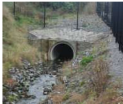
New R151 culvert exit in Bettystown.
