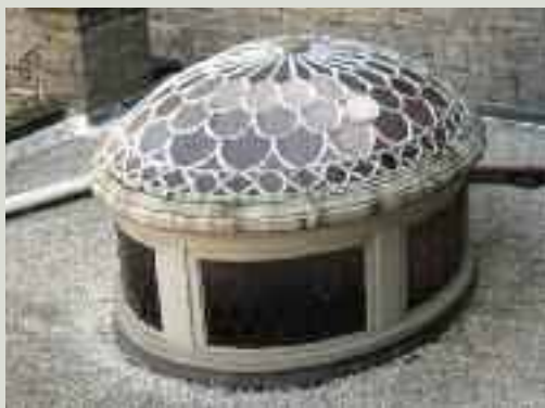
Historic skylights and lanterns, such as this fine example, should be well-maintained but are rarely suitable for thermal upgrading
