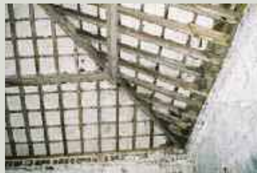
A roof with largely intact lime mortar parging applied to the underside of the slates. Parging has an insulation value in itself and helps to reduce air-blown water infiltration
