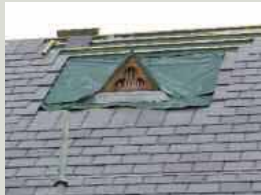
A special detail was used to deal with the small additional height that resulted from adding insulation to the roof build-up; stone blocks were added under the reinstated cast-iron gutter
