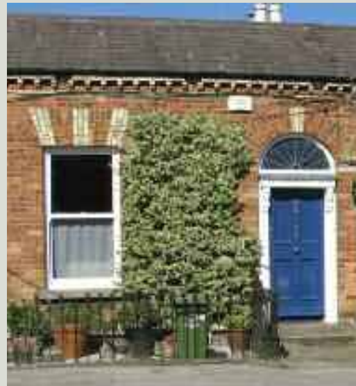
A typical brick-fronted, nineteenth-century house with solid masonry walls, single-glazed sash windows and slate roof
