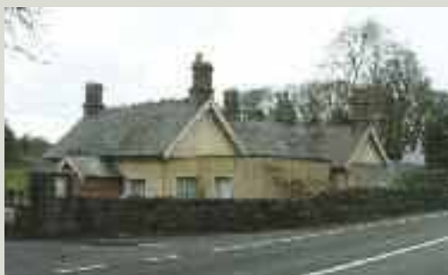
Cottages prior to refurbishment
