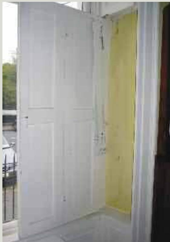
A well-sealed shutter lining
