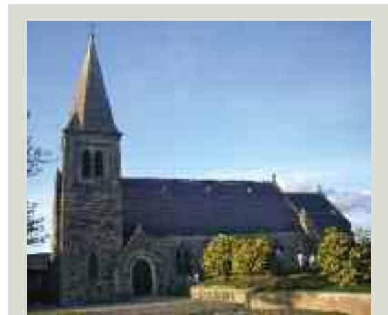
A nineteenth-century church with spire. The roof has been re-slatted and insulated and the walls re-pointed
