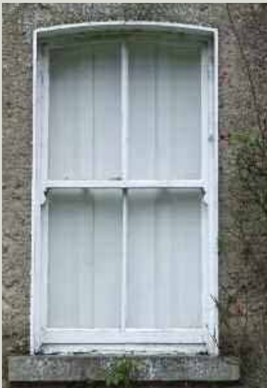
Working timber shutters: the interior of the shutter boxes could be lined and sealed to reduce air leakage. Any new linings should not prevent the shutters from folding back into the shutter box when not in use
