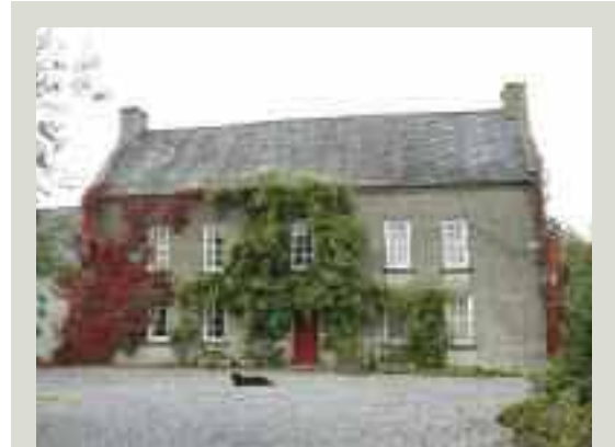
A typical traditional farmhouse, built of stone and finished in lime render, with a slate roof and timber windows
