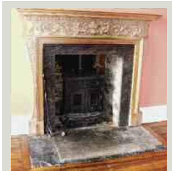
Wood-burning stoves can be efficient but in a traditional building they should generally only be fitted into non-decorative fireplaces. Historic grates and fire surrounds should not be damaged or removed in order to fit a stove
