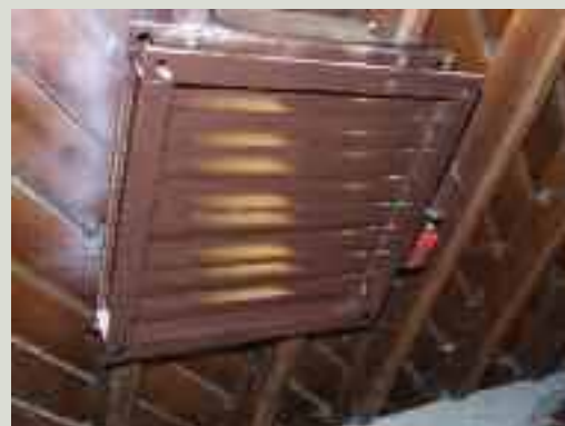
While re-slating, the opportunity was taken to put the original ceiling vents back into working order. The vents are mechanically controlled to allow the users to alter the amount of ventilation as required
