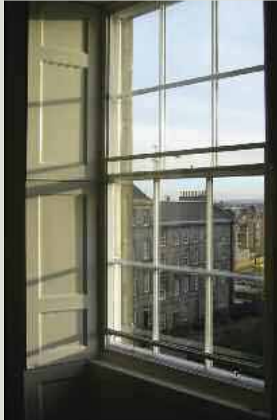
Carefully designed bespoke secondary glazing installed as part of Changeworks' Energy Heritage project (Image © Changeworks)
