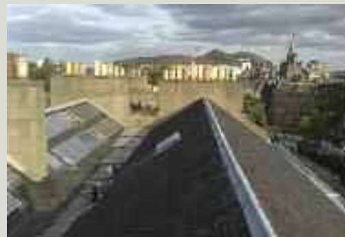
A roof valley may be an appropriate place to locate solar thermal or photovoltaic panels provided that the orientation of the roof is appropriate. This image shows solar panels installed in hidden roof valley as part of Changeworks' Renewable Heritage project (Image © Changeworks)
