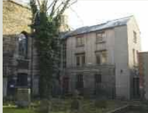
This new extension to the rear of the church provides necessary office accommodation and comprises two storeys built on top of the ruins of the original vestry
