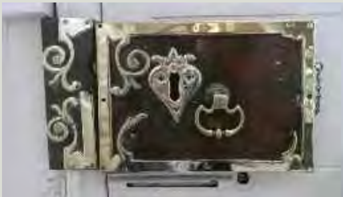
Some historic door furniture may be difficult to use, such as this lock case in Fitzwilliam Square. It should nevertheless be retained in-situ and an alternative means of opening the door provided
