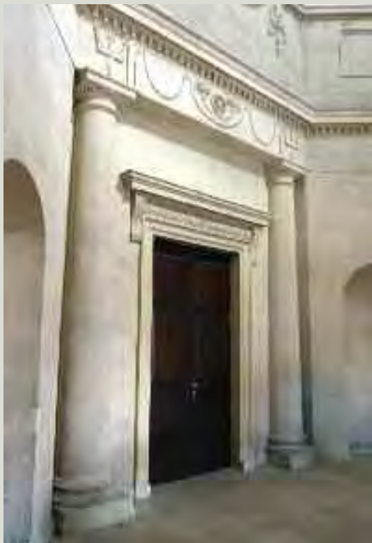
Historic doorcases are often generous in proportion and frequently provide good colour contrast to aid in their location. When door knobs are difficult to use, it may be possible to ensure the door remains open
