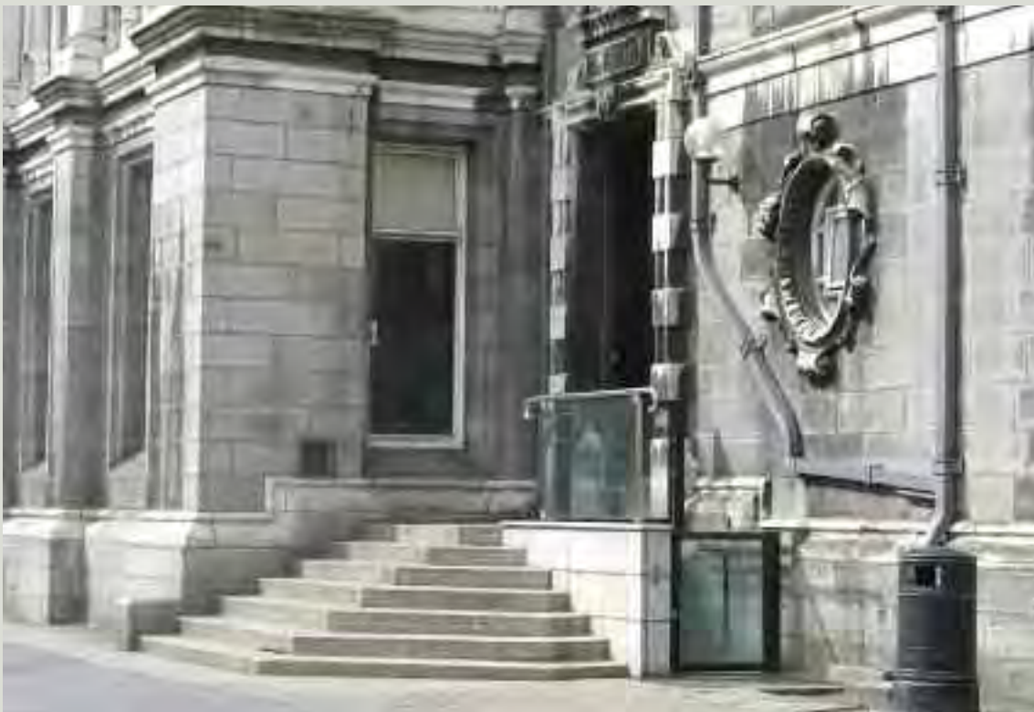
Mechanically operated short-rise lift systems using high quality materials can be sensitively integrated if well designed
