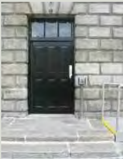
When carrying out the alterations to raise the landing and provide wheelchair access to this building the existing outward opening double doors which had been fitted in the 1980s were removed and a single new door and fanlight based on the design of a pre-existing door nearby was installed, thereby providing sufficient space at landing level for a chair to turn. An important consideration was the relationship of the new landing level to the door frame and other elements of the façade
