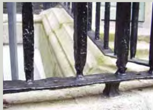
Bars do not necessarily need to be replaced when they have wasted at their base. Unless their condition is compromising the integrity of the ironwork, they can be left in place
