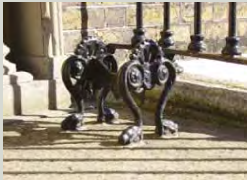
Eighteenth- and nineteenth-century boot scrapers are still a common feature of houses across Ireland
