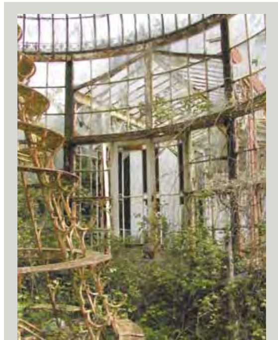
This finely-made circular conservatory was designed and erected at Castlebridge House, County Wexford by James Pierce of Mill Road Iron Works, Wexford. In addition to its iron structure, it contains a 10-tier iron display stand for plants at its centre
