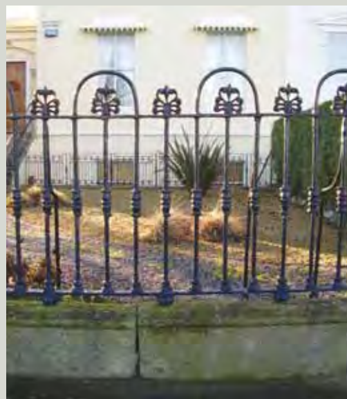
Early nineteenth-century railings incorporating fashionable Neo-Classical decoration such as cast iron collars, husks, and anthemion (honeysuckle) finials
