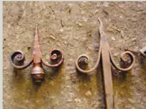
While modern welding techniques are not ideally suited to traditional ironwork, a skilled craftsperson may be able to apply modern welding to repairs to a level that is visually acceptable. The finial on the left has been forge welded and hammered down to a point, while the finial on the right has been electric arc welded and then hammered into a point in the traditional way
