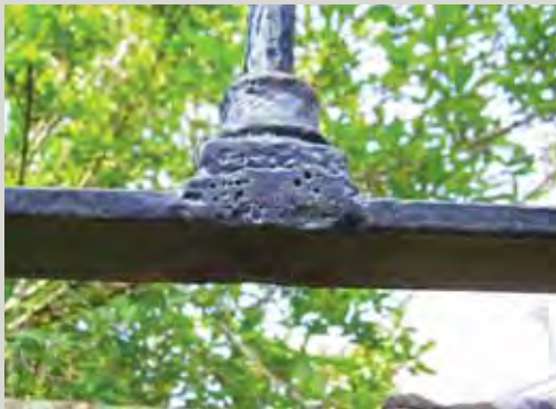
Paint cannot fill holes. Casting flaws such as those pictured above should be filled to prevent water becoming trapped and causing corrosion to develop
