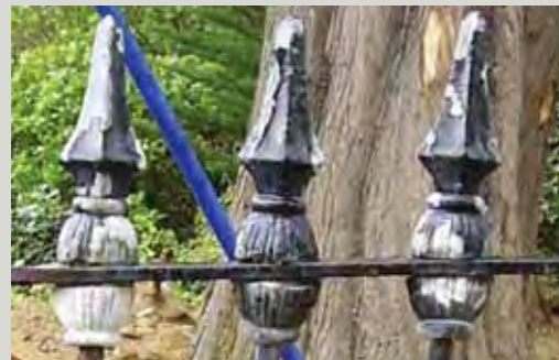
Aluminium is not an appropriate substitute for grey cast iron
