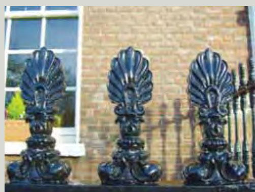
Mid nineteenth-century railings with wrought iron bars and rails, and decorative cast iron finials and husks
