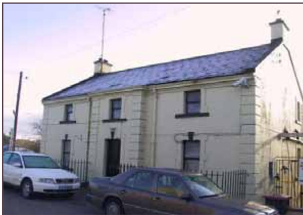
Fig. 41: North elevation of the hotel.
