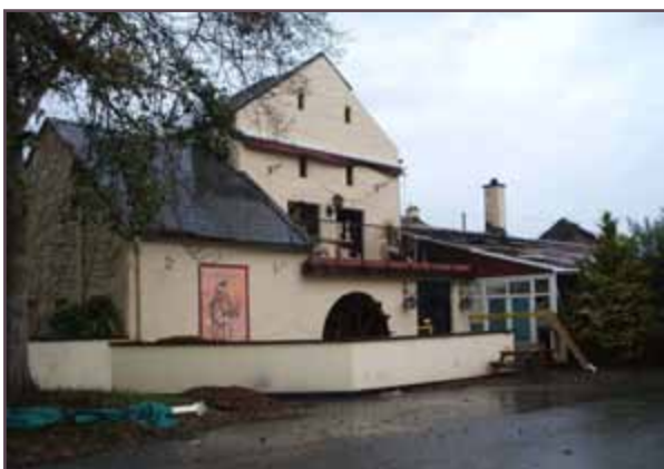
Fig. 53: View of the of mill building.
