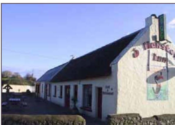
Fig. 37: The north elevation viewed from the car park.
