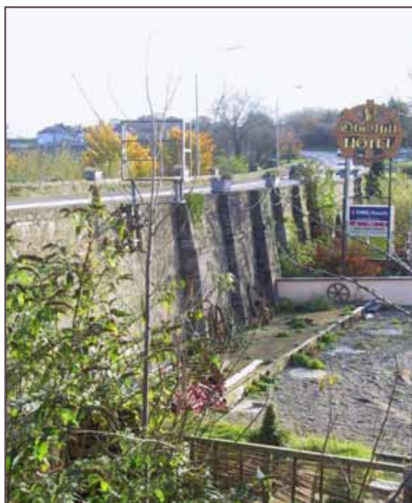
Fig. 34: The view of the bridge from road level.
