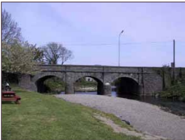
Fig. 27: View of the bridge from the west.
