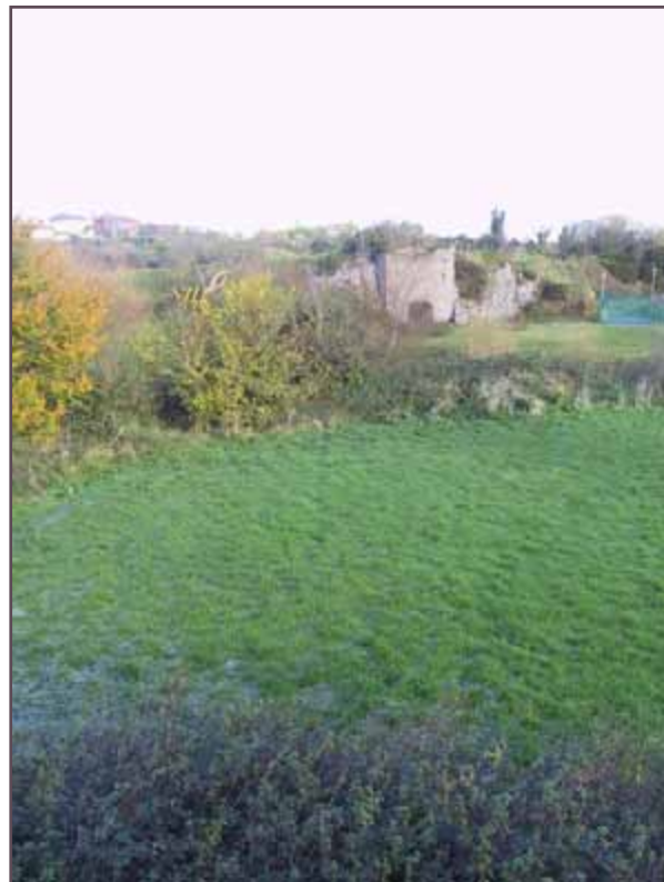
Fig. 18: View of the lime kiln, St. Mary's and Nanny.
