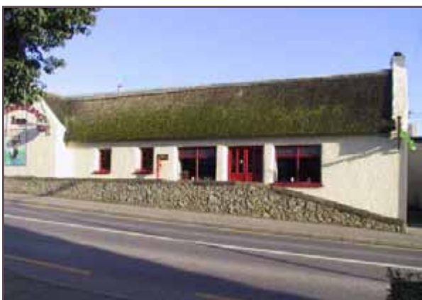
Fig. 36: The west elevation of the pub from the road.
