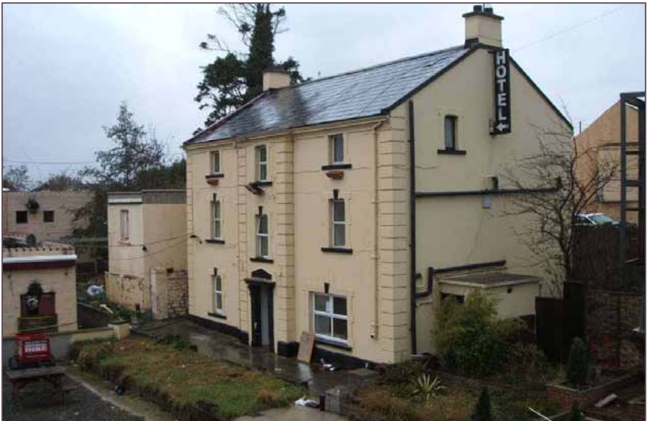
Fig. 57: View of the mill house from the bridge.
