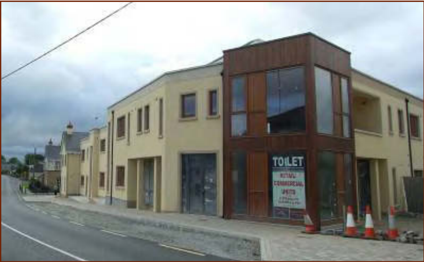
Fig.10a: New development on Kilglass Road
