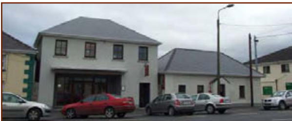
Fig.16: Main Street, new buildings, south side
