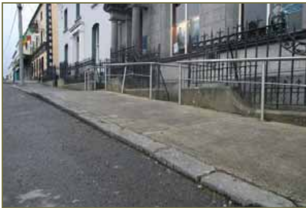
Fig. 38, 39: Oliver Plunkett Street, steps to terrace houses, railings and kerbs in front of the National Bank
