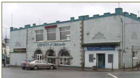
Fig. 9: Market-house east side
