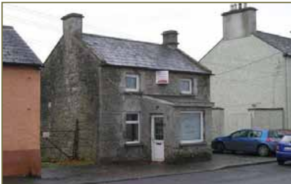
Fig. 23,24: Cogan Street; former RIC Barracks, stone house
