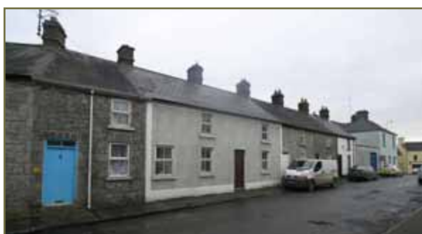
Fig. 27: Cloughan Street, terrace of houses on the east side
