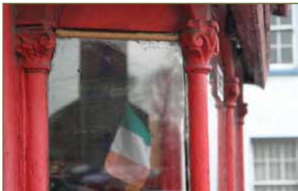
Fig. 14,15: Herbstreit Shopfront and window detail
