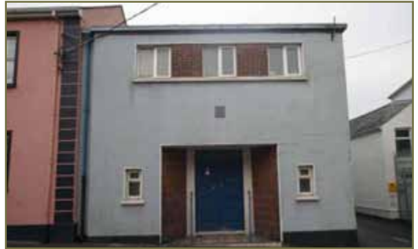
Fig. 31: Church Street, former Masonic Hall
