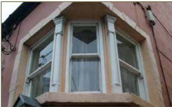
Fig. 29,30: Church Street, Farrelly's pub, elevation and first floor corner window
