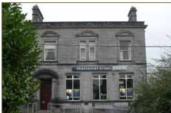
Fig. 33, 34: Oliver Plunkett Street, terrace houses (west), National Bank building (east)
