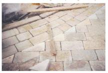
New stone paving being laid to a curve.
