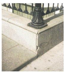
Thin stone veneer is prone to damage and cracking.
