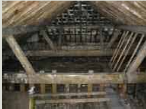
An eighteenth-century re-roofing of a tower house using imported deal
