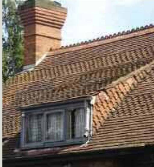
The nineteenth century saw a resurgence in the use of terracotta tiles as part of a revived interest in handmade building materials. Clay tiles allowed the introduction of colour and decoration at roof level, creating a whole new aesthetic
