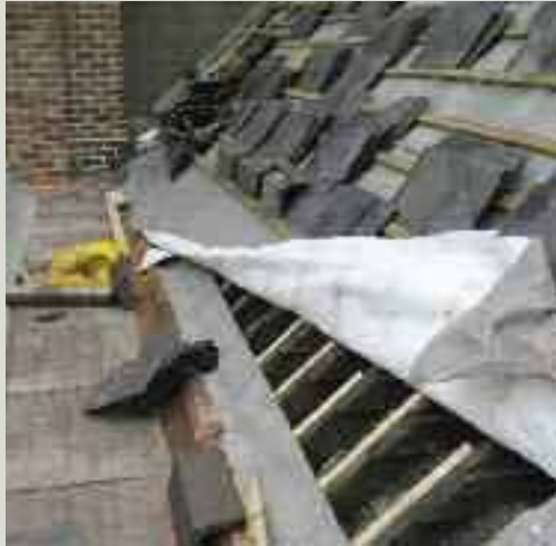
Re-lining a valley gutter in copper. Splice repairs were required to the ends of rafters where the previous valley had leaked over a significant length of time, causing decay of the timber structural elements below
