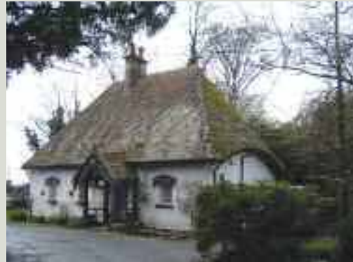
A gate lodge with a decorative clay-tiled roof, having striking curved elliptical eaves and a patterned use of plain and scalloped tiles. Overhanging branches and the proximity of large trees have tended to promote extensive moss growth on part of the roof
