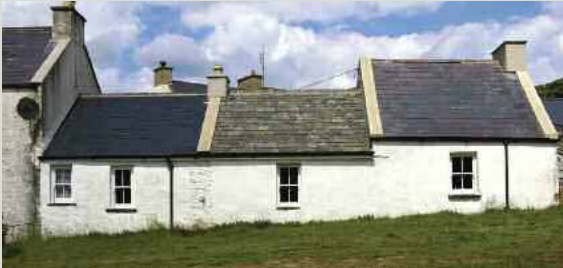
Most buildings using stone roofing slate are distinguishable by their simple gable-ended roofs. Hipped profiles, dormer windows, and valleys are difficult to achieve because of the large and somewhat unwieldy nature of the stone slate
