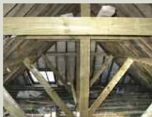
These rafters were originally undersized for their span and had deflected, causing slates to lift or slip, and thus allowing water to enter the roof space. To correct the problem, this additional support structure was added during roof repair works
