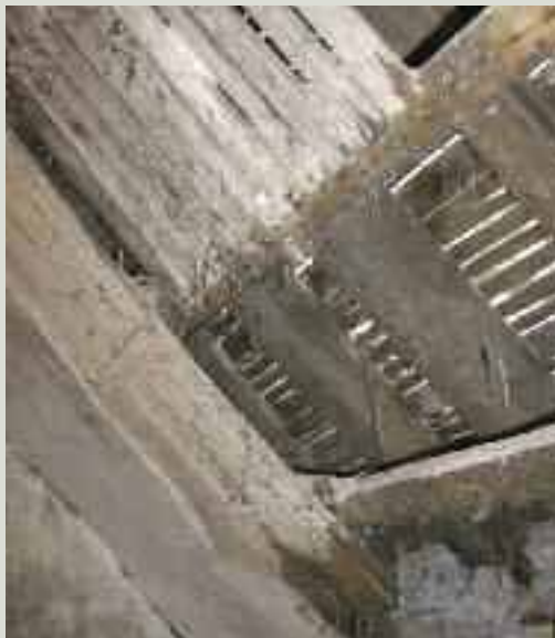
The recent discovery, within a later roof space of part of the former medieval friary in Ennis, of closely spaced riven laths fixed onto covered-over rafters substantiated the presence of an earlier structure within the historic fabric
