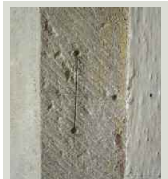
A mason's mark carved into a finished piece of stone. This is a simple mark of a type common in the thirteenth century. Later masons' marks were more elaborate and often in relief. Note the diagonal tooling
