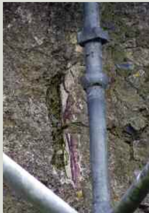
Rare surviving painted decoration on mediaeval plasterwork can be seen on this part-concealed pilaster (Image courtesy of the Office of Public Works)
