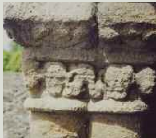
Carved sandstone, showing weathering. Sandstone was widely used for carving because it was relatively soft and easily worked. Some high crosses and Romanesque detailing were carved in sandstone
