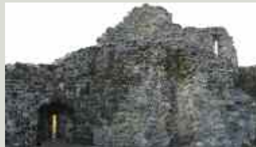
A repair to a town wall using new stone where the wall had been damaged or robbed. In this case, the new stone was sourced from a quarry 8 km away and, in the course of time, will weather in
