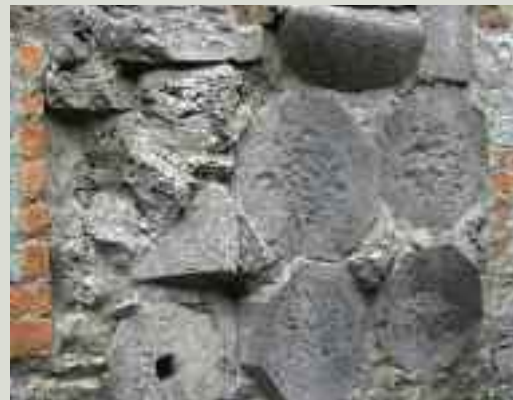
Earlier carved stone was often reused in the construction of later masonry walls. In this example an opening was blocked up using parts of a disassembled column from the adjacent ruined friary
