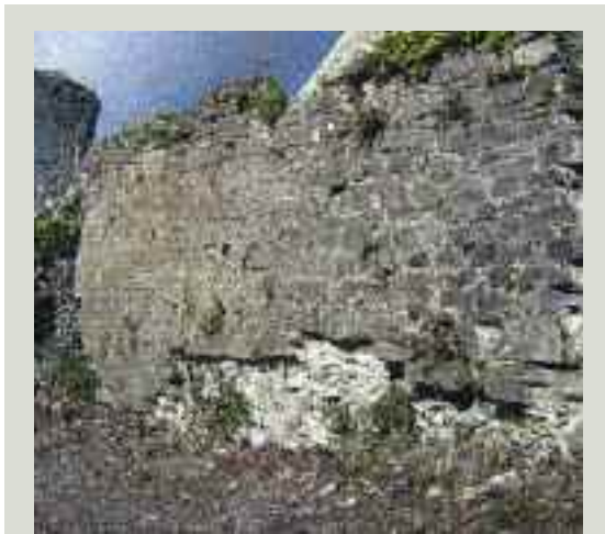
Stone has been robbed from this section of a town wall and probably used to build other masonry structures nearby
