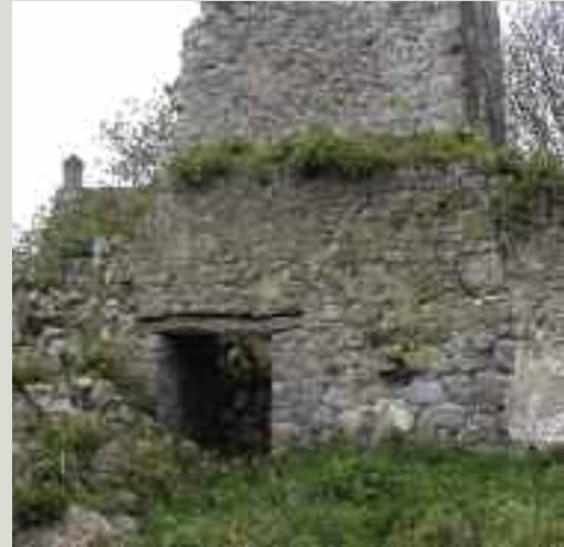
The condition of the surrounding masonry is important in the survival of timber lintels. If the wall top or pointing is poor, water will lodge on top of the timber lintel and cause decay
