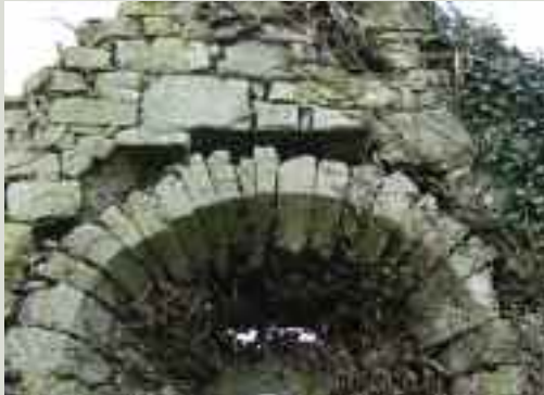
Arch over a window. Note the damage done by the improper removal of ivy which pulled out the smaller packing stones and has left the arch vulnerable
