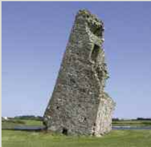
A leaning structure which has stood for many years in this position
