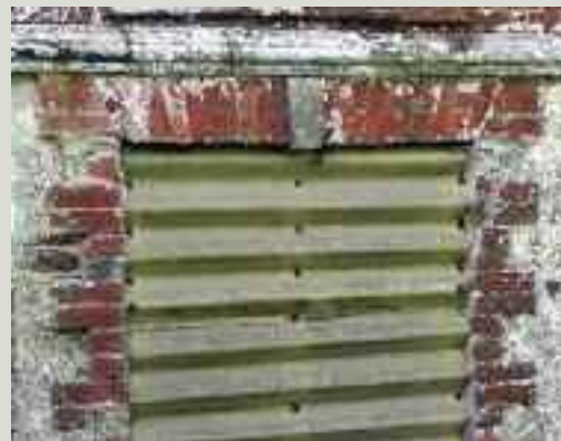
A flat arch constructed of brick with a limestone keystone
