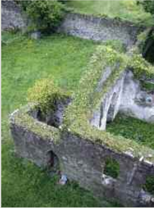
Wall tops are particularly vulnerable to being colonised by grass and seedlings. While some of these plants may be relatively harmless, others such as ivy and saplings should not be allowed to take root
