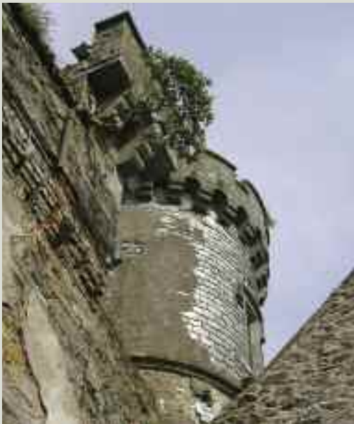
While more commonly found as a roofing material, slate was also used as a cladding material for exposed walls, gables and chimney stacks. The slates found in slate-hanging are often rare examples of native Irish slates which, because of their small sizes, were often replaced on roofs by Welsh slates
