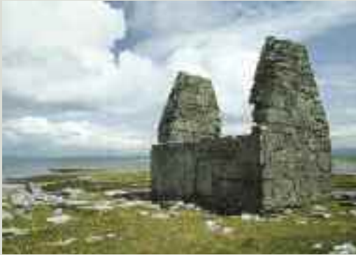
The stark simplicity of the early mediaeval oratory of Temple Benan on Inishmore shows a sophisticated use of local stone including large thin blocks of limestone laid on edge
