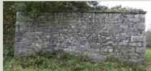
Uncoursed random rubble. Note the large quoin stones at the corners which give strength to the structure
