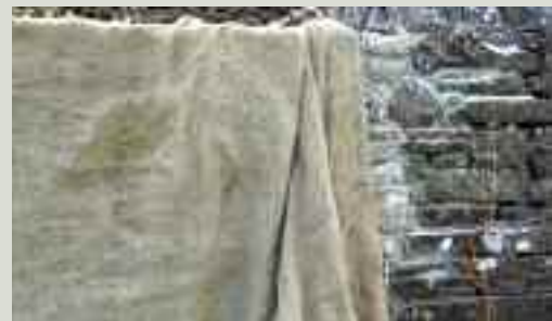
Protective hessian on masonry work is far more effective than plastic sheeting and can be reused many times
