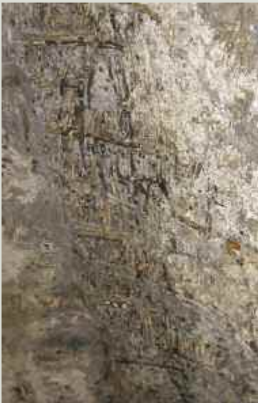
In this example of wicker centring on the underside of a vault, not only the imprint of the wickerwork but also parts of the original wicker matting itself have survived embedded in the mortar layer
