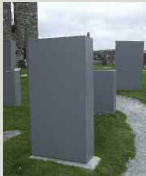
Graveyard with headstones protected by plywood casings in advance of conservation works to the adjacent structure
