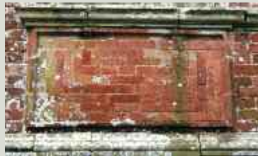
Fine early handmade bricks together with limestone dressings were used in the construction of Palace Anne, County Cork built in 1714
