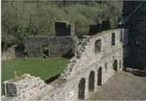
Flaunching, a sloping area of mortar, has been applied to the raking surface and also to the upper surface of this wall on which a mat of vegetation is beginning to grow
