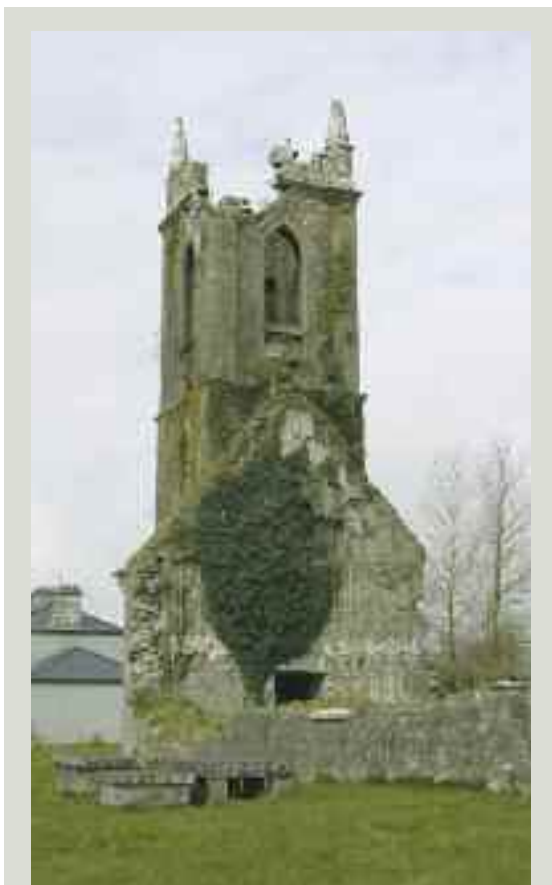
Ruins are often found in isolated areas and a structure such as a tower may be the tallest in its locality making it vulnerable to lightning strike. The tower of this ruined church was struck by lightning which destroyed the corner pinnacle
