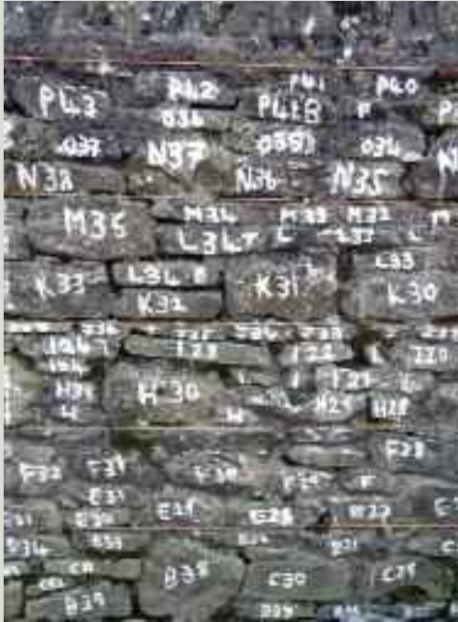
Masonry wall with stones numbered to allow for accurate rebuilding. The strings are stretched across the length of the wall to mark the wall at vertical intervals to ensure joints are kept at original thickness when rebuilding
