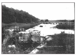
Fig.3: Lawrence photograph from the late nineteenthcentury showing the limestone piers to the flood-gates, weir, bridge and the original mill building beyond, without the addition of the brick chimney. Courtesy of the National Library of Ireland.
